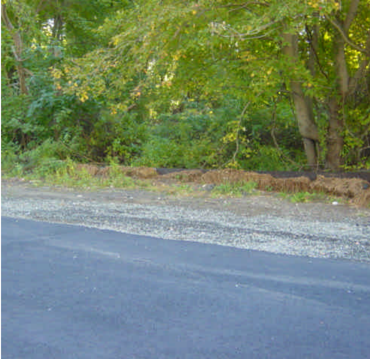
Area near sta. #1015-1020 has been repaved as part of final restoration. Some hay bales remain in one area near sta. #1017. Silt fence should be removed but haybales can remain.
