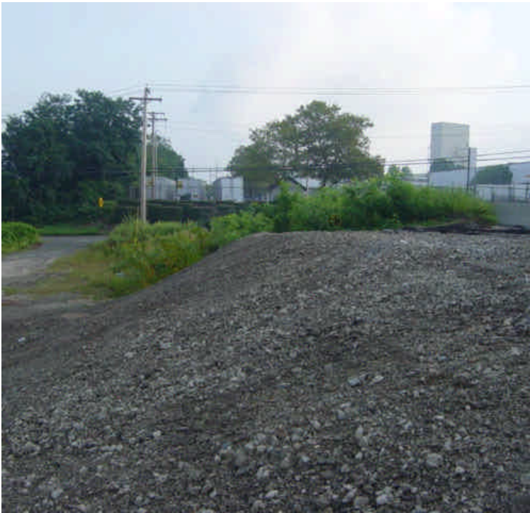
Area near sta. #1080 was re-graded several weeks ago and remains exposed. Continue to monitor and permanently stabilize the area as soon as possible.
