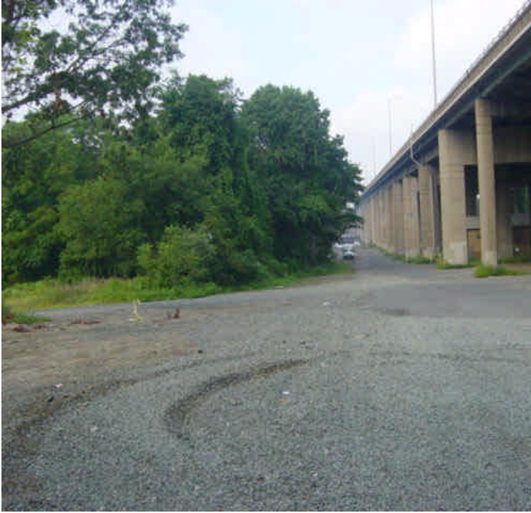
The area near sta. #15-20 remains backfilled with crushed stone and is generally stable. Final restoration is on-hold pending a planned DOT drainage project.
