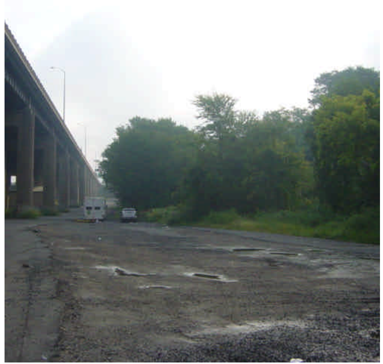
The area near sta. #15-20 remains backfilled with crushed stone and is generally stable. Final restoration is on-hold pending a planned DOT drainage project.
