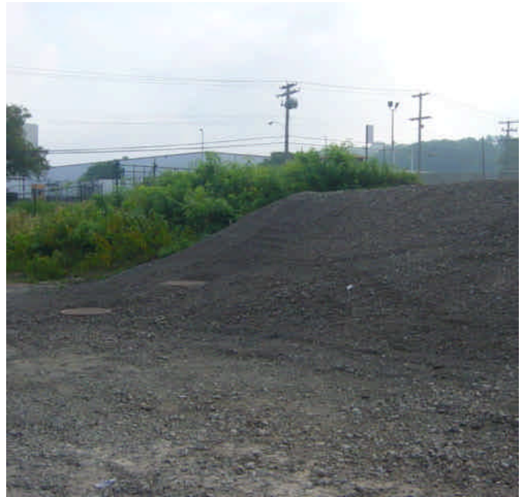
Area near sta. #1080 was re-graded several weeks ago and remains exposed. Continue to monitor and permanently stabilize the area as soon as possible.
