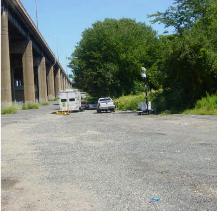
Electrical contractor was on site at vault #1. The areas have been backfilled with crushed stone and are generally stable. Final restoration is on-hold pending a planned DOT drainage project.
