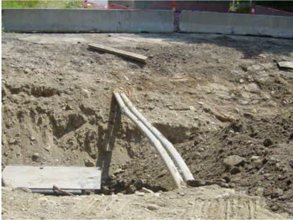
Both circuits have been tied-in to the HDD work near sta. #1020. Backfilling was underway at the time of the inspection.
