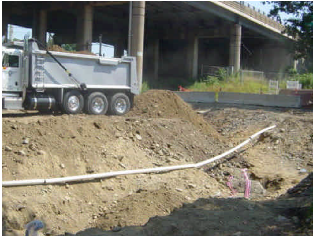
Both circuits have been tied-in to the HDD work near sta. #1020. Backfilling was underway at the time of the inspection.
