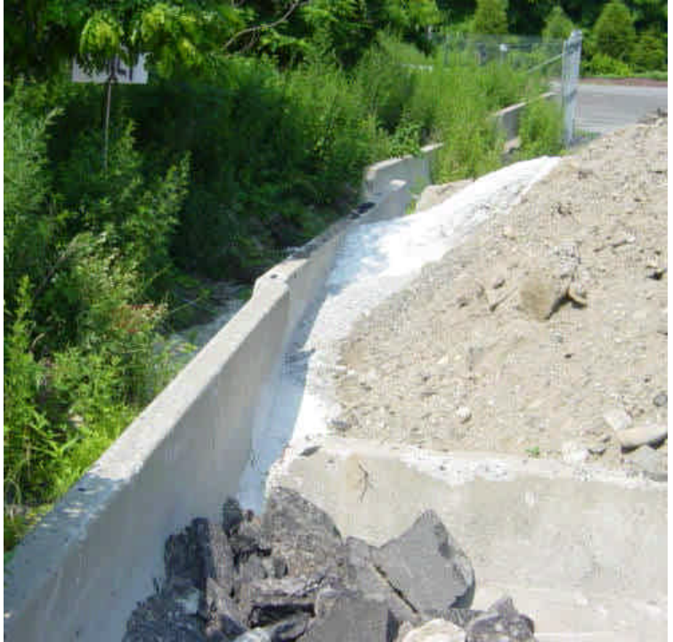
Evidence of what appears to be several concrete washouts were observed near the material storage bunkers. Slurry material flowed out the back of the bunker and towards the entrance to the yard where it eventually cured. No concrete work associated with the project was ongoing when the washouts occurred. It is unclear whether the washouts are project related.
