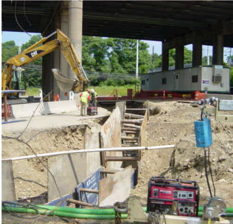
Trenching continues near sta. #1020 to tie-in to the HDD work.
