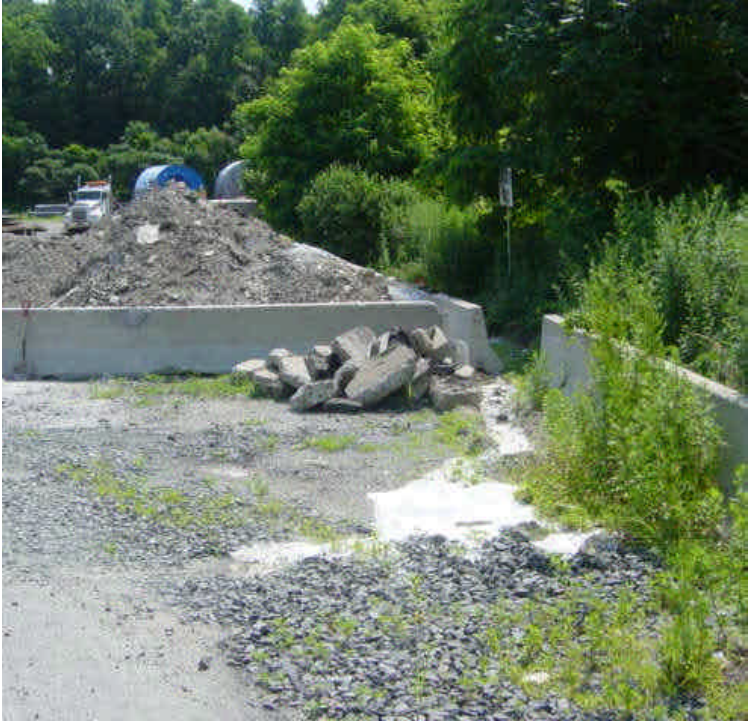
Evidence of what appears to be several concrete washouts were observed near the material storage bunkers. Slurry material flowed out the back of the bunker and towards the entrance to the yard where it eventually cured. No concrete work associated with the project was ongoing when the washouts occurred. It is unclear whether the washouts are project related.
