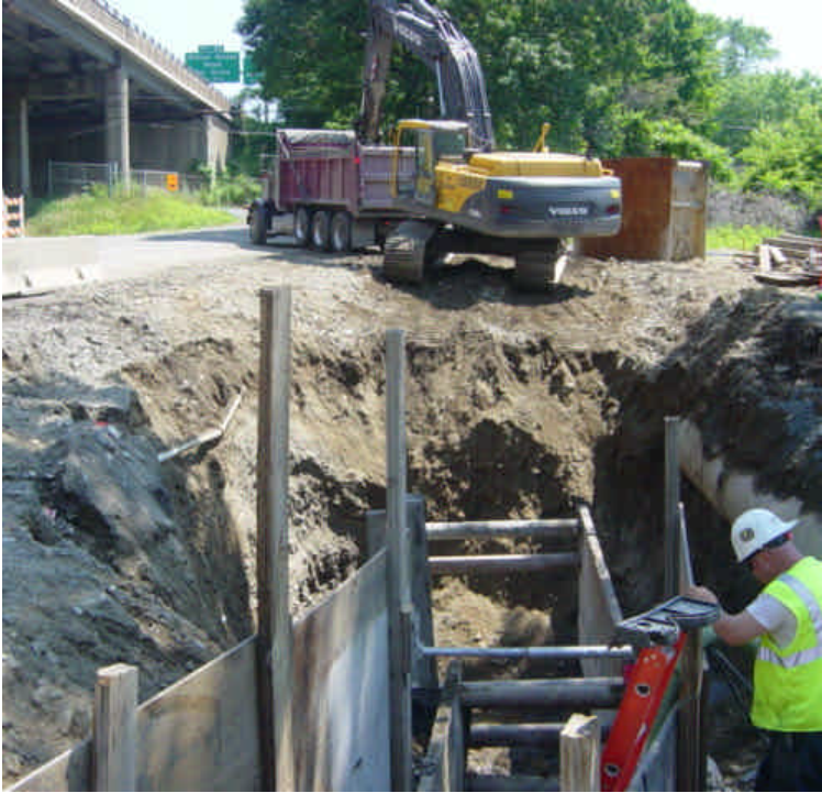
Trenching continues near sta. #1020 to tie-in to the adjacent HDD work.
