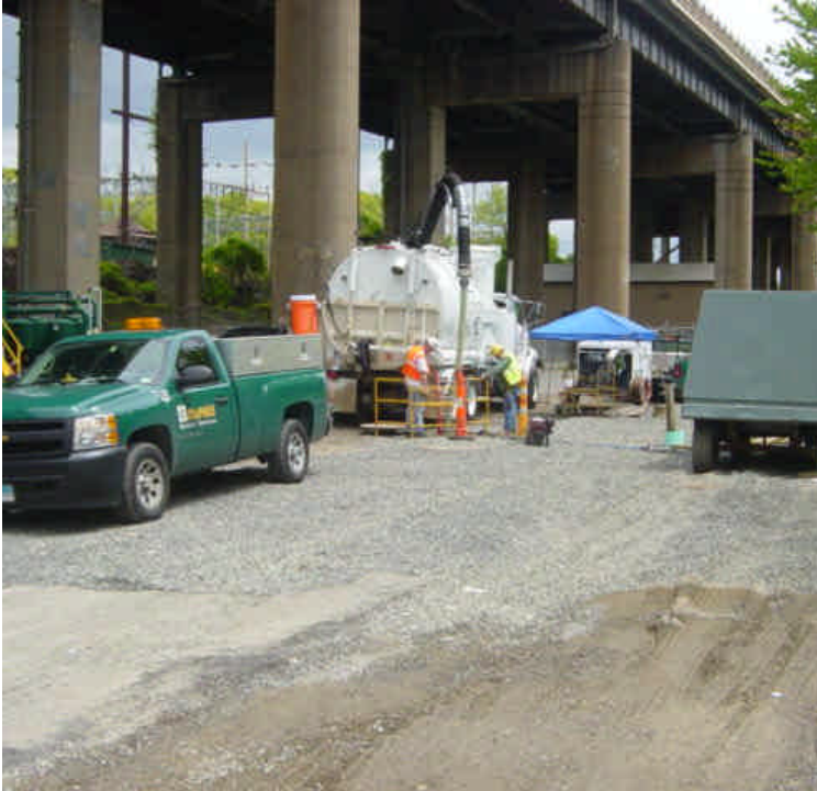
Electrical contractors were on site proofing the lines at vault #1.
