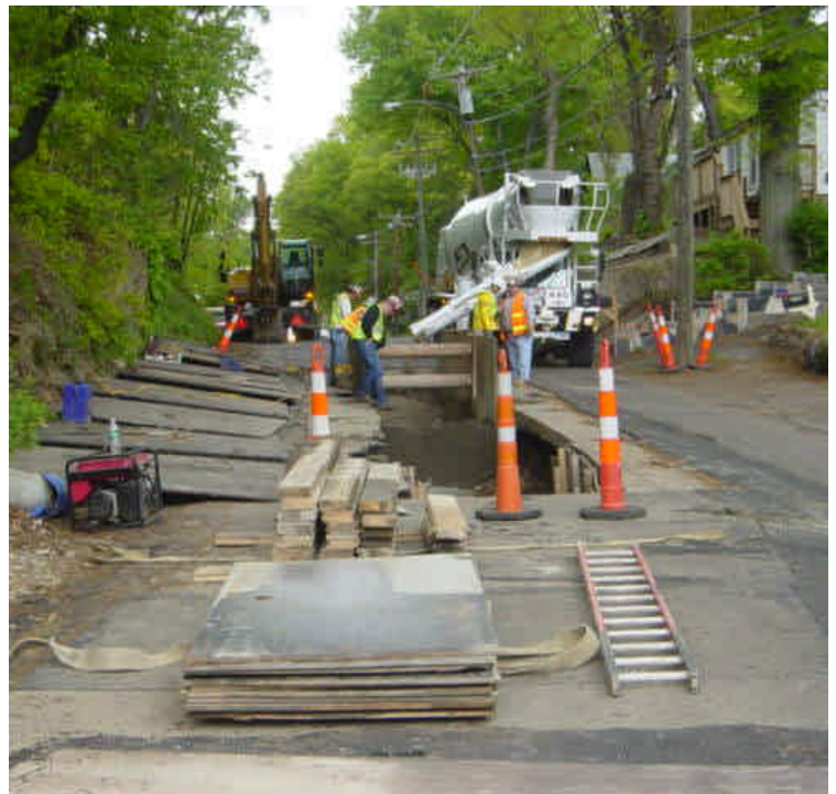
Backfilling was ongoing near sta. #1030-1031.
