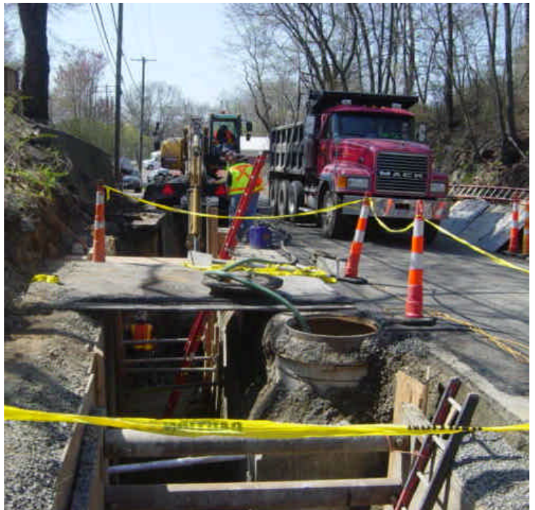
Trenching continues along Naugatuck Avenue near sta. 1030-1032.
