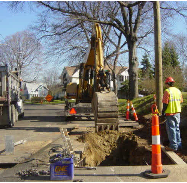
Trenching continues along Naugatuck Avenue near sta. #1042-1044.
