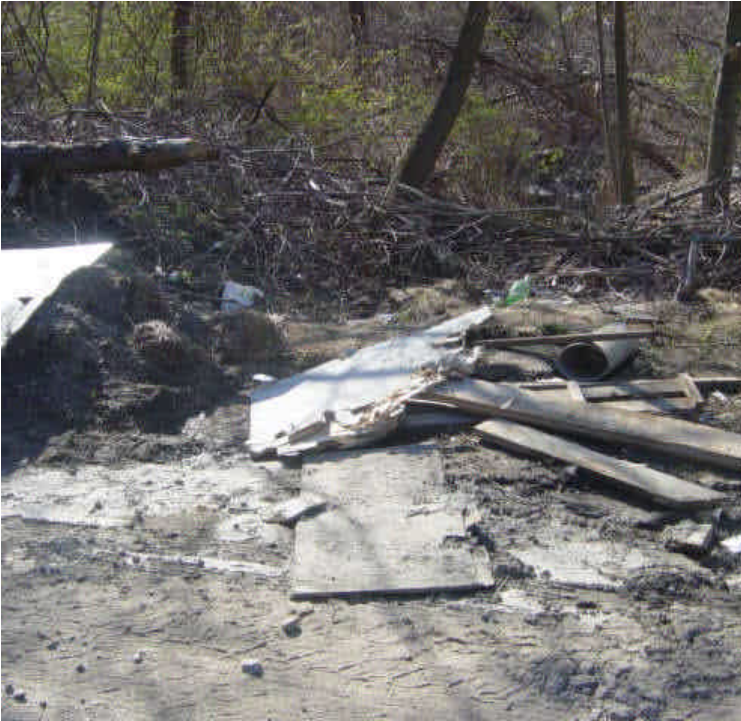
Debris material has been placed near the drainage swale along the south side of the staging area. The haybales are deteriorating and a resource area is adjacent. This area should be cleaned up as soon as feasible and controls should be evaluated.
