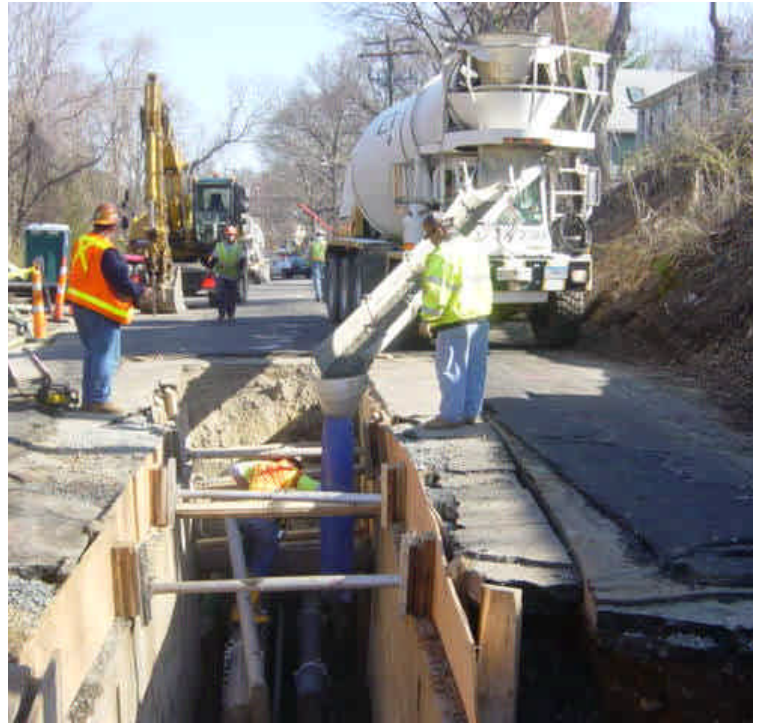
Backfilling was underway near sta. #1031-1032.
