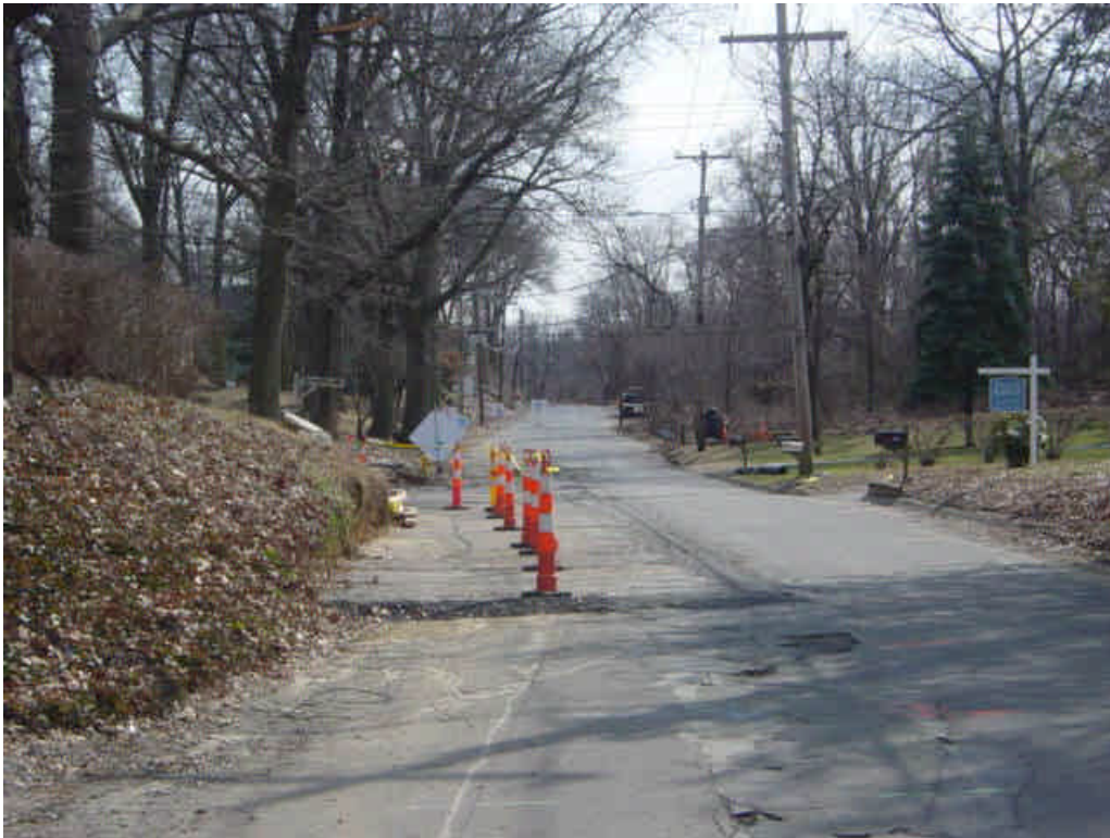
Water meters were recently relocated along Naugatuck Avenue by the City of Milford.
