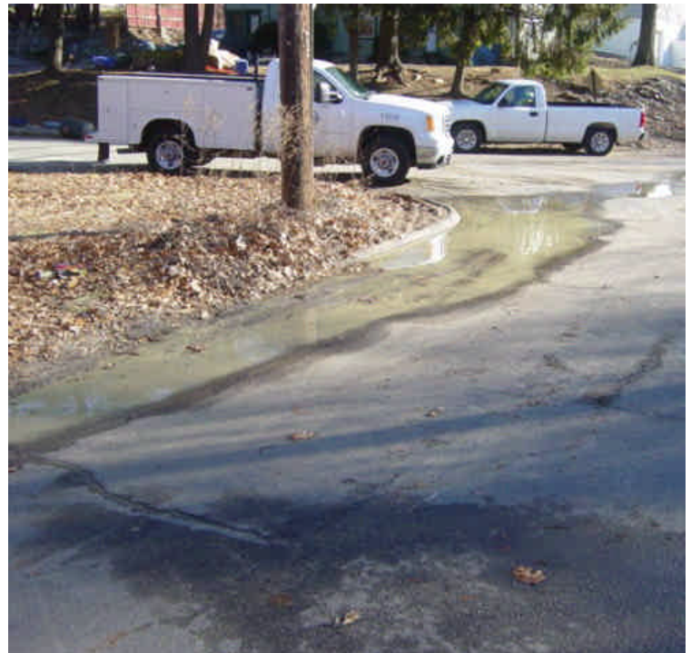
Trenching and backfilling activities continue along Naugatuck Ave near sta. #1037 to 1038. At the time of the inspection the trench was being backfilled. Concrete slurry had mixed with the groundwater which was being pumped down the street towards a plugged catch basin near sta. #1034. The runoff was ponding along the roadway. The supervisor was informed of the problem and the crew agreed to vacuum out the catch basin at the end of the day. Evaluate dewatering methods and ensure they are in compliance.
