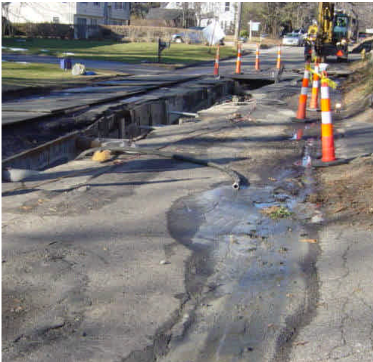
Trenching and backfilling activities continue along Naugatuck Ave near sta. #1037 to 1038. At the time of the inspection the trench was being backfilled. Concrete slurry had mixed with the groundwater which was being pumped down the street towards a plugged catch basin near sta. #1034. The runoff was ponding along the roadway. The supervisor was informed of the problem and the crew agreed to vacuum out the catch basin at the end of the day. Evaluate dewatering methods and ensure they are in compliance.
