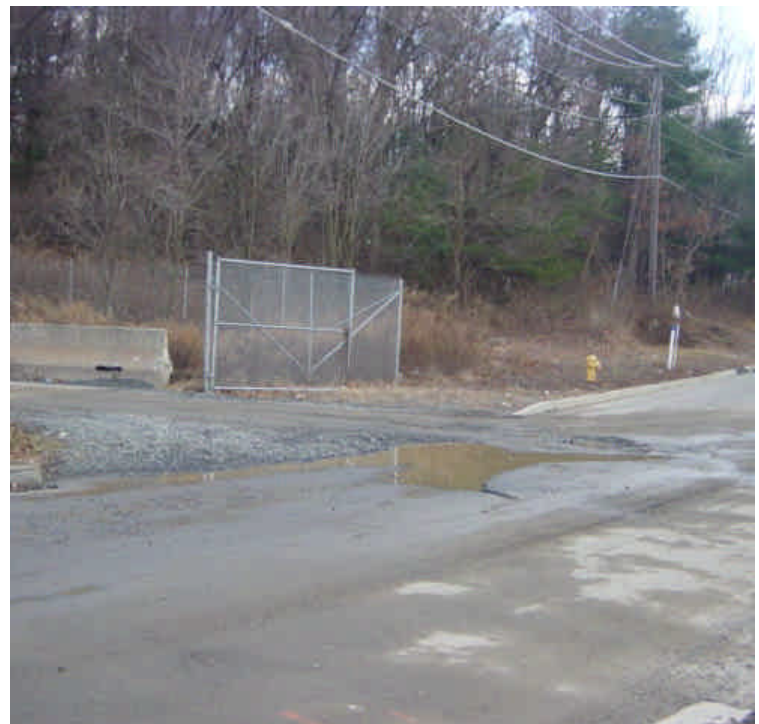
The Shelland Street lay-down yard was muddy and sediment tracking was observed from the entrance of the yard. Stone may need to be refreshed here.
