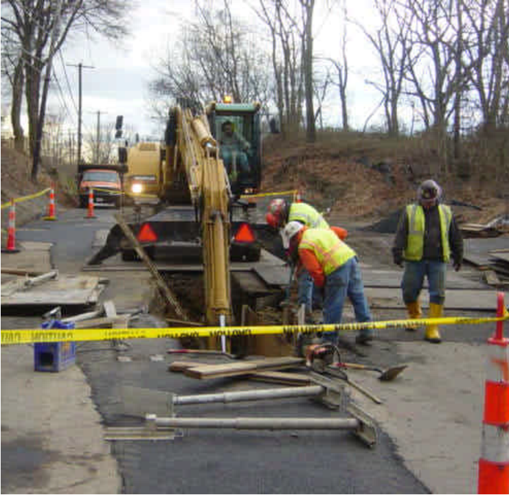
Trenching activities continue along Naugatuck Ave near sta. #1032 to 1033.
