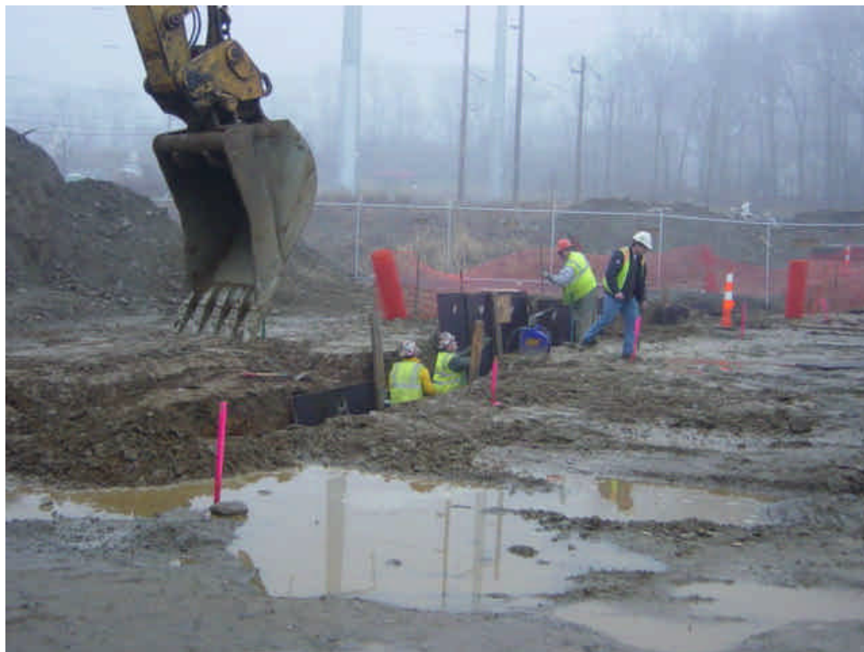
Trench work has resumed near the East Devon substation, from station #1114-1117.
