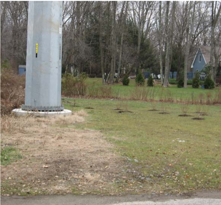
Salem Rd: An additional view of restoration efforts and plantings near structure #3910/24097.
