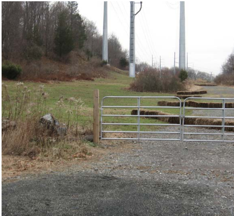
Old Ln: A view of the controls and restoration efforts near structure #4015/24202.
