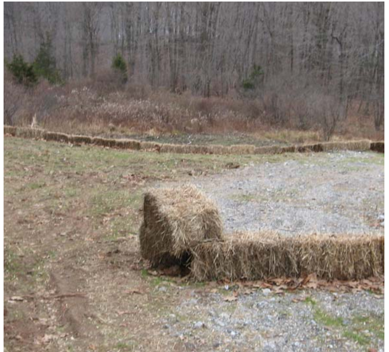
Gaylord Mtn Rd (Hamden): Haybale controls have been added along the slope near structure #3993/24180. Soils appear stable in this area at this time.
