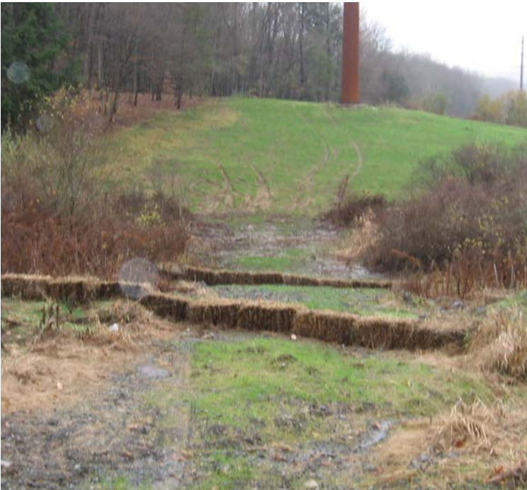
Old Ln (Hamden): A view of the restoration efforts and controls that remain functional near structures #4012/24199.
