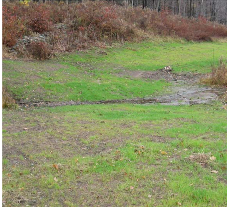
Pease Rd/JCC: No further scouring/sedimentation to the intermittent stream channel has been observed here. Haybale controls are recommended along the stream channel as a proactive measure.
