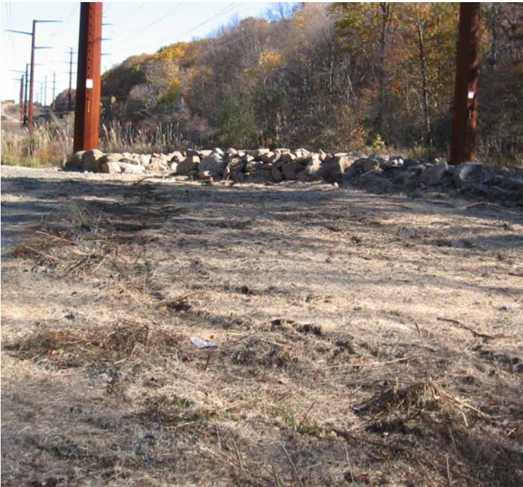
Hatfield Rd (Bethany): A view of the restoration efforts near structures #3979/24166.
