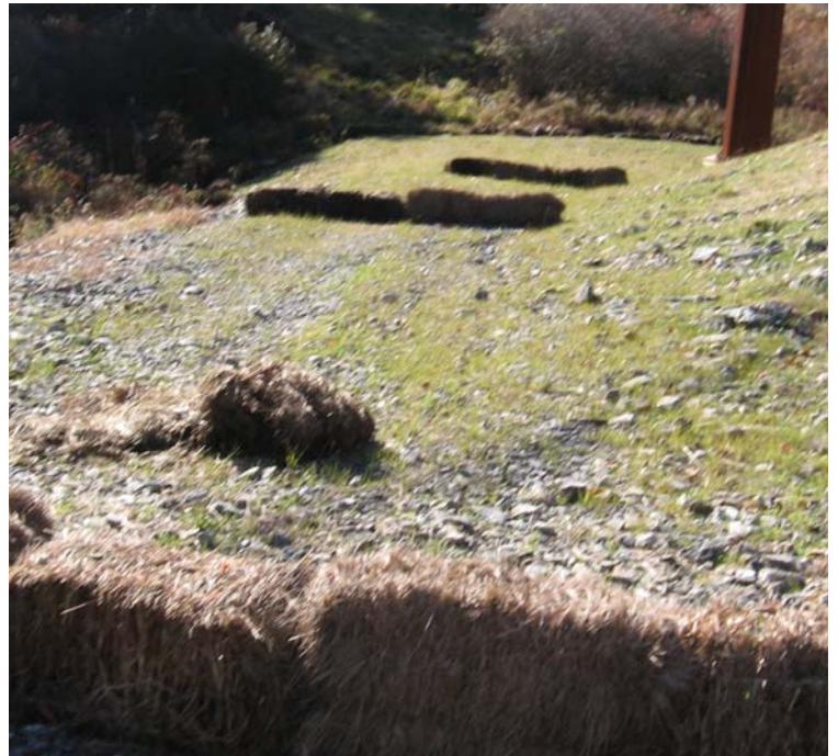
Litchfield Turnpike: A view of controls and restoration efforts near structure #3960/24147.
