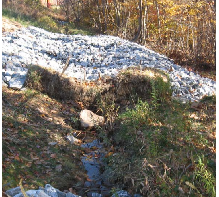
Gaylord Mtn Rd: An additional view of stone and haybale controls.
