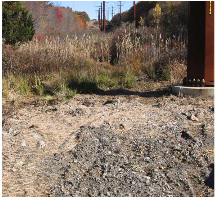
Hatfield Rd: A view of the wetland restoration efforts near structures #3979/24166.
