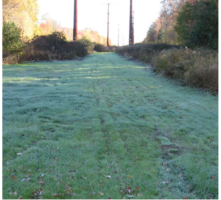
Russell Ave: An additional view of the restoration efforts within the access road.
