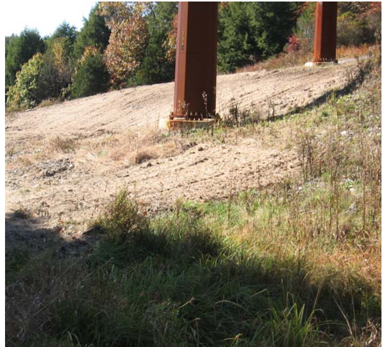
Hatfield Rd (Bethany): A view of the restoration efforts near structures #3971/24158.
