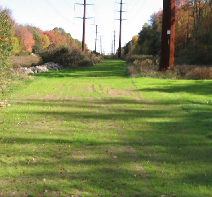
Treat Ln (Orange): A view of the vegetative cover within the access road. Final stabilization efforts have been achieved here.
