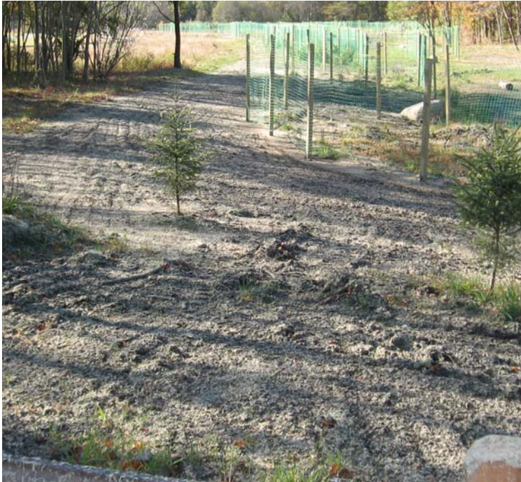
Eisenhower Park (Milford): Hydro-seed has been applied to the exposed soils around the mitigation area.
