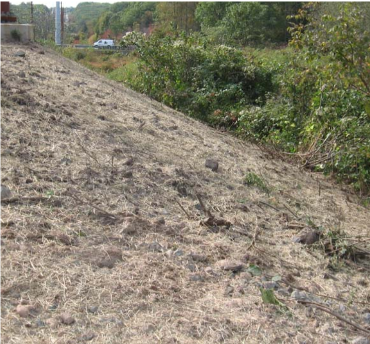
Willow St: View of the crane pad restoration efforts near structures #4009/24196.
