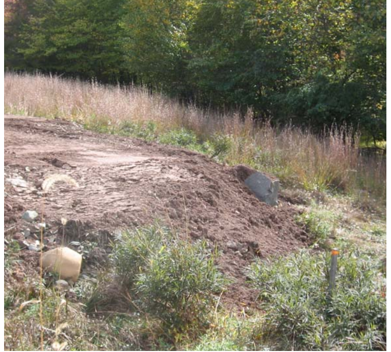
Dogburn Rd south: Exposed soils remained upgradient of a wetland following crane pad reclamation near structure #24082.
