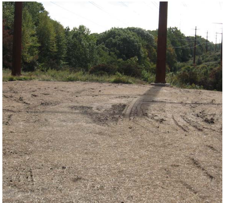
Tom Swamp: View of the restored crane pad near structures #3994/24181.
