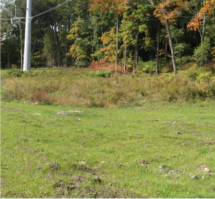
Rimmon Rd/B'Nai (Woodbridge): Good vegetative cover has been noted within the cleared wetland. Final stabilization has been achieved in this section.
