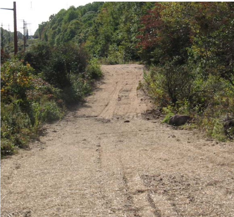
Tom Swamp (Hamden): View of the restored access road.
