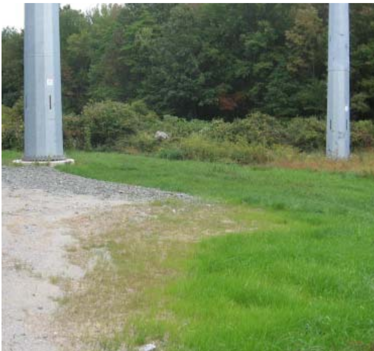
Manville Rd: A view of the restoration efforts near structures #3916/24103. This area has achieved final stabilization.
