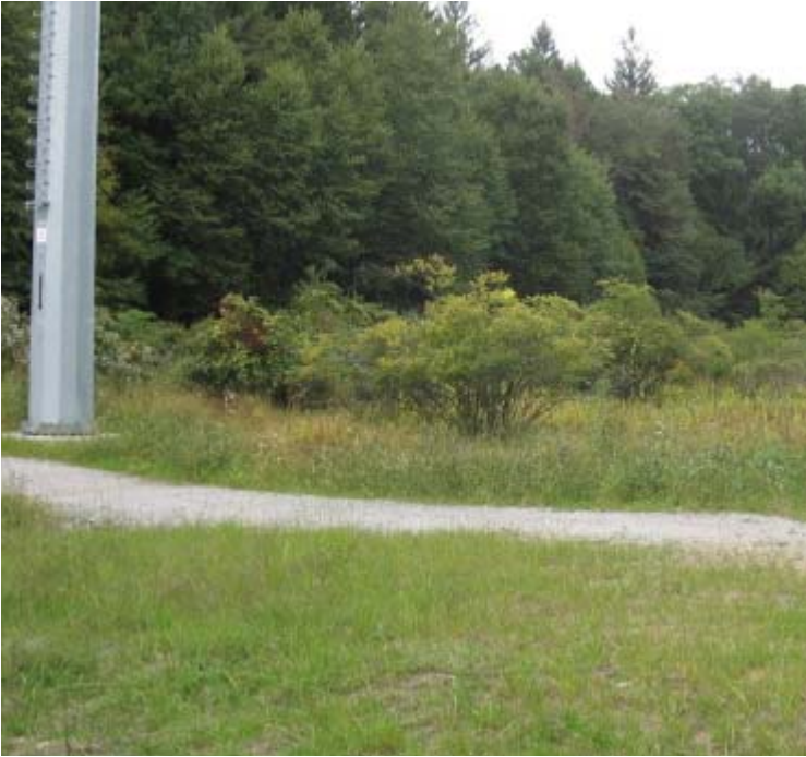
Clearview Ln: A view of the restoration efforts near structure #3903/24090. A permanent wetland crossing remains here as permitted. Final stabilization efforts have been achieved in this area.
