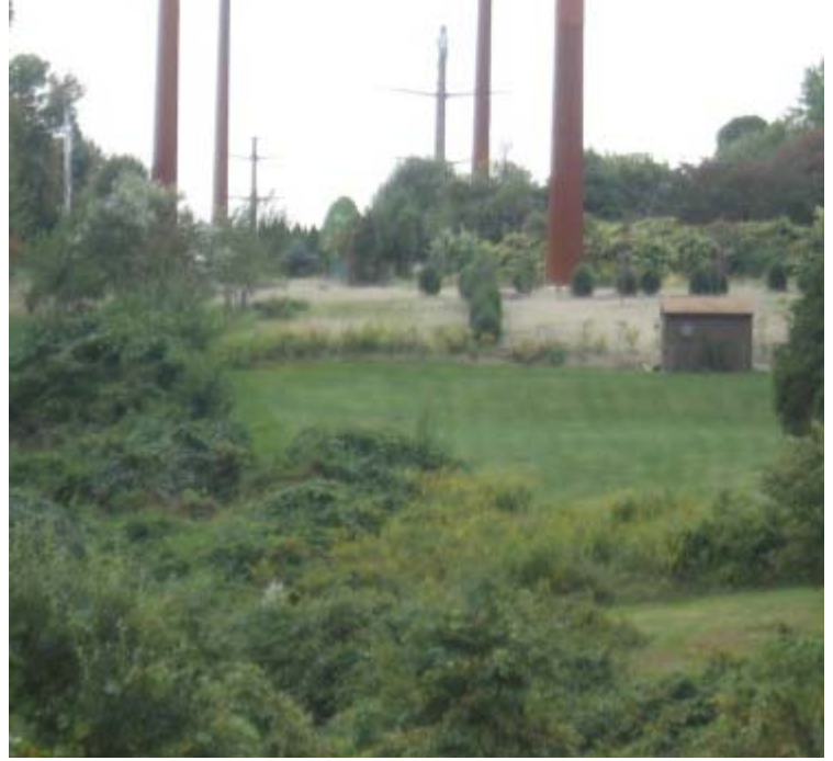
Rt 34: A view of the restoration efforts and plantings off Saddle Ridge road near structures #3884/24071.
