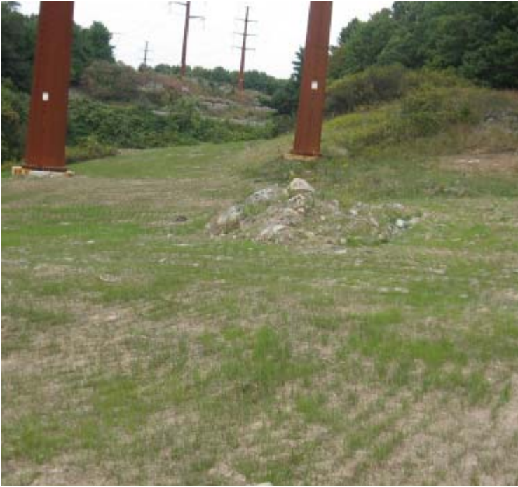
Rt 34 (Orange): Vegetative growth continues within the restored access road and crane pad near structures #3887/24074.
