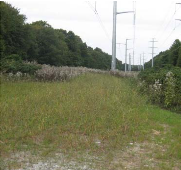
Clearview Ln (Woodbridge): A view of the restored upland access road near structures # 3901/24088.
