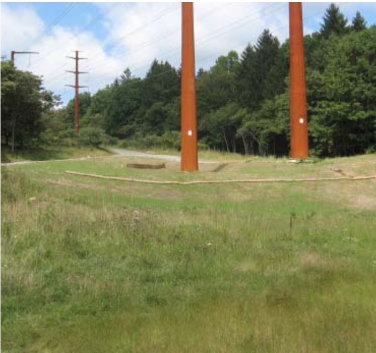
Dogburn Rd (Orange): Restoration efforts near structures # 3890/24077.
