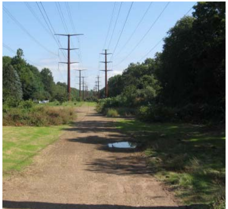
Treat Ln: An additional view of the restoration efforts in this area.
