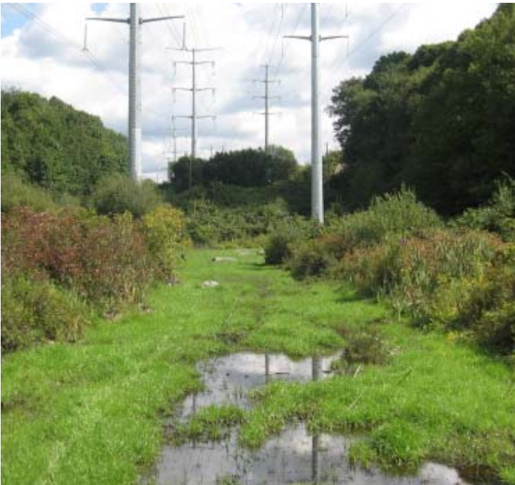
Rimmon Rd/B'nai Jacob: A view of the restored access road near structures # 3923/24110.
