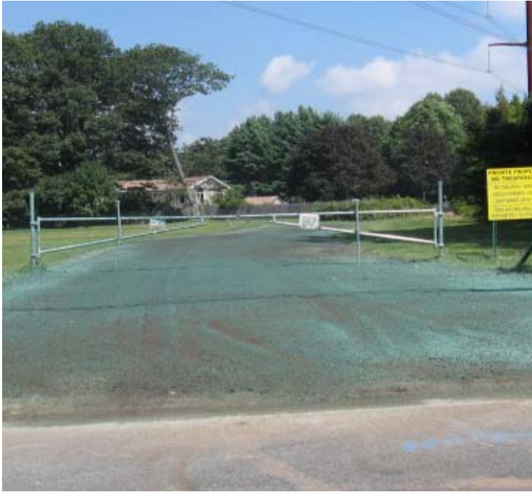
Treat Ln (Orange): View of restoration efforts. Hydro-seed was applied here.
