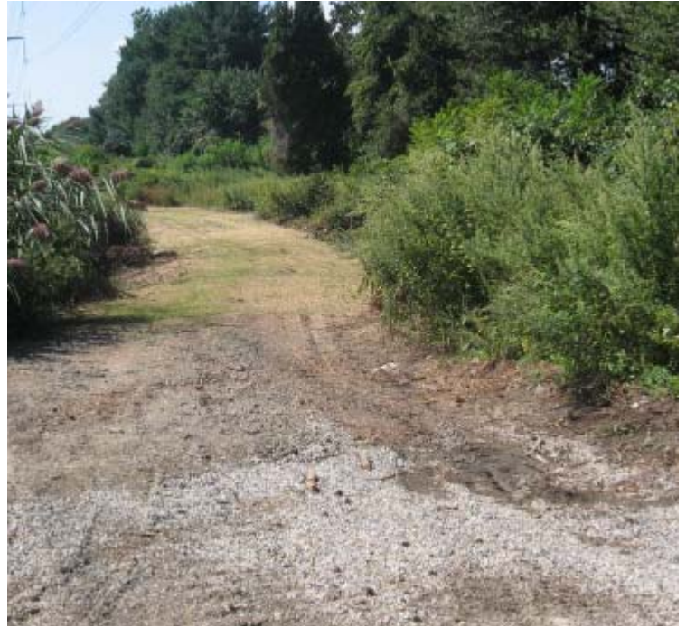
Treat Ln: The permanent wetland crossing here has been stabilized with mulch and seed. Vegetation growth is evident.
