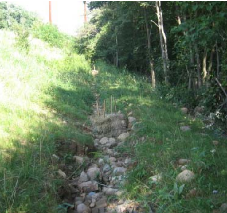
Gaylord Mtn Rd (Hamden): Haybales have been placed in the swale to help control stormwater run-off.
