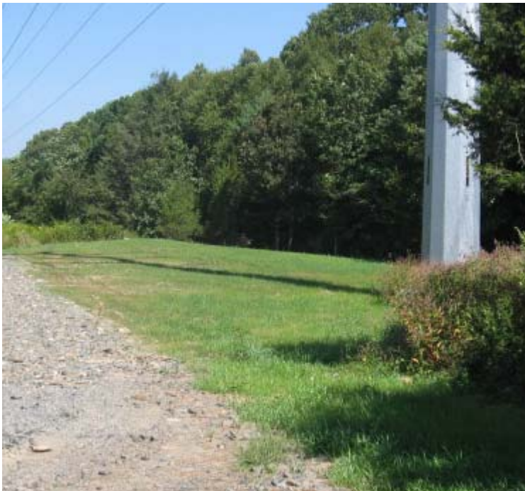
Cowpath Ln (Woodbridge): Vegetation covers approximately 70% of the former crane pad area near structure #3940.
