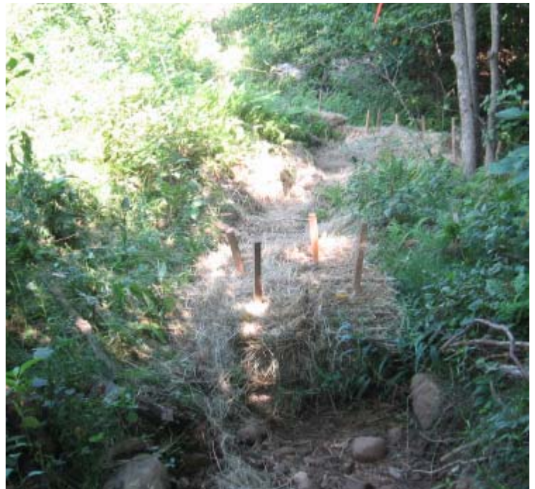
Gaylord Mtn Rd: An additional view of the haybales added to the Swale.
