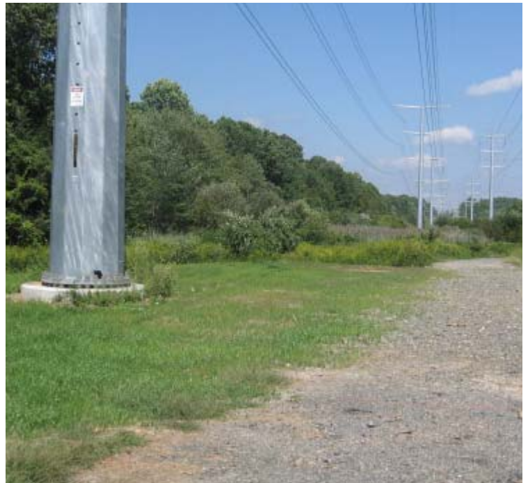
Cowpath Ln: Vegetation covers approximately 70% of the former crane pad area near structure #24127.
