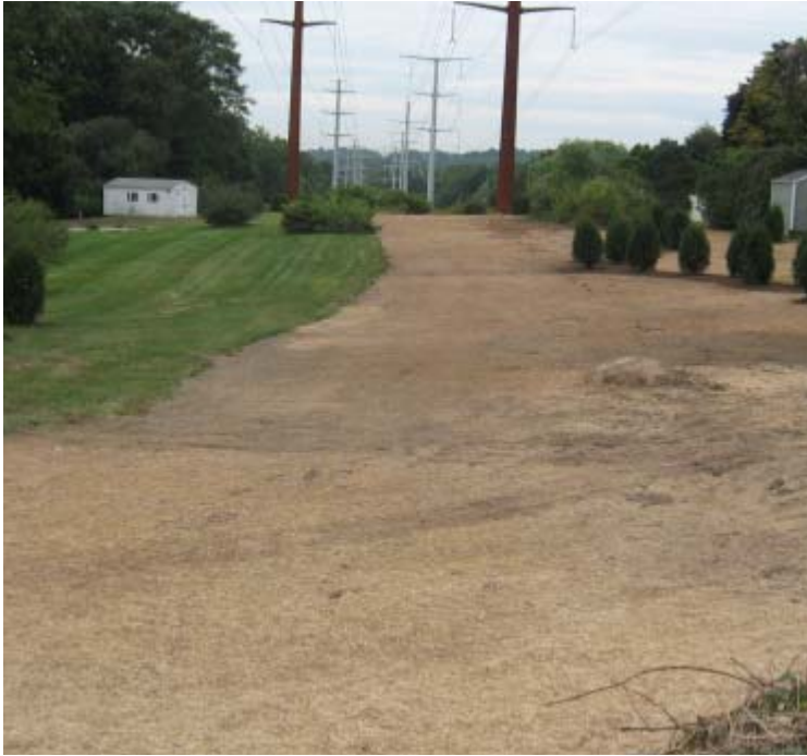
Ridge Rd (Orange): A view of restoration efforts in this area.
