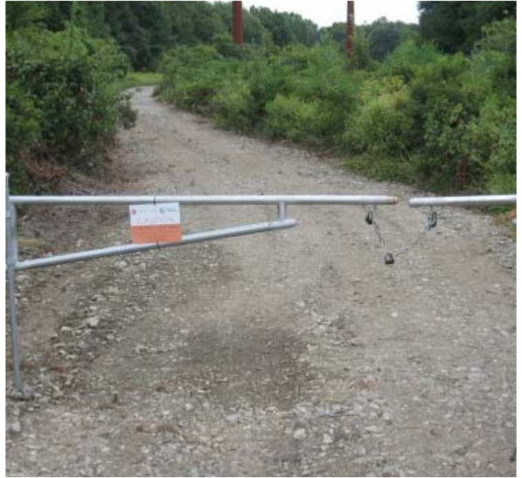
Pine Tree Dr (Orange): A permanent stone access Rd has been installed in the wetland here, as permitted.
