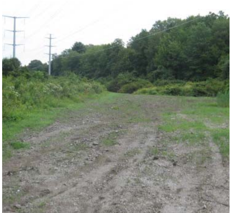
West River St: Exposed soils remain in the upland portion of the ROW where the access road was removed.
