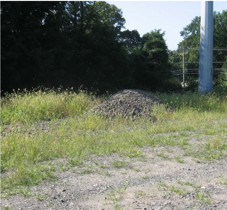
Wheelers Farm Rd: A spoil pile remains in the ROW near structure #3830.
