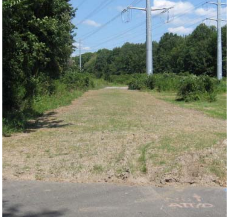
Manville Rd (Woodbridge): A portion of the access road has been restored. The remaining portion is permanent and will remain in the wetland, as permitted.
