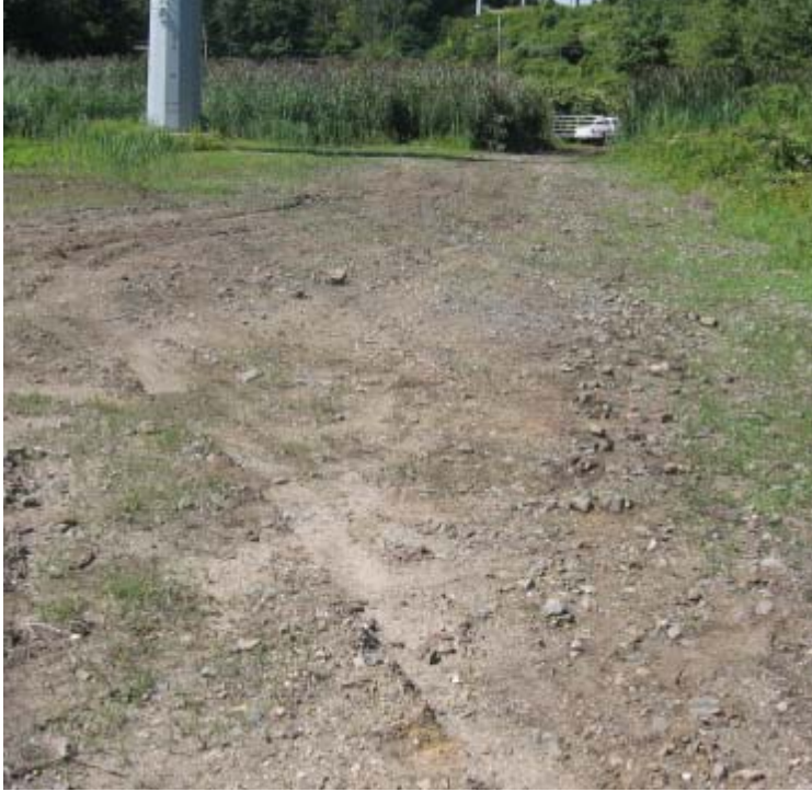
West River St: Exposed soils remain in this area.
