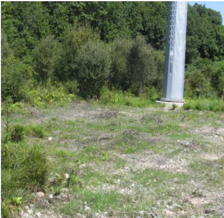
B'Nai Jacob (Woodbridge): A view of crane pad reclamation.
