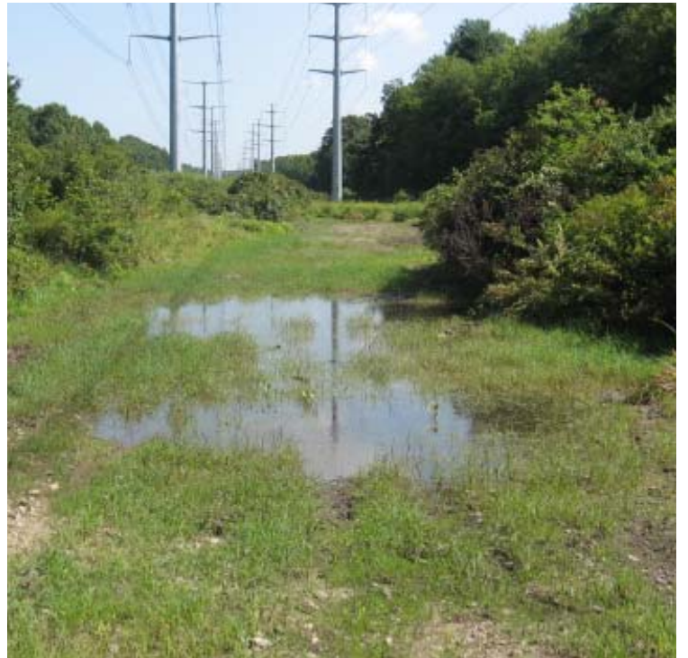
West River St (Milford): Vegetative growth has been noted in some areas of the reclaimed access road.
