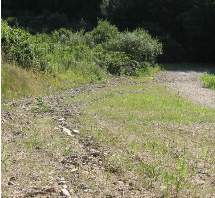
East Rutland (Milford): Some scouring is evident on the slope of the former crane pad.
