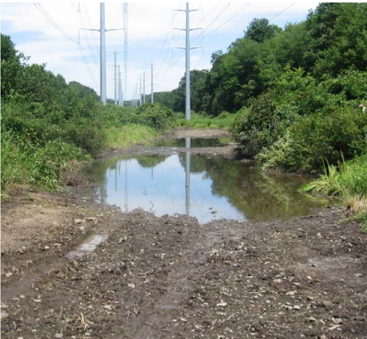
West River St: An additional view of where the access road has been returned to the original grade.
