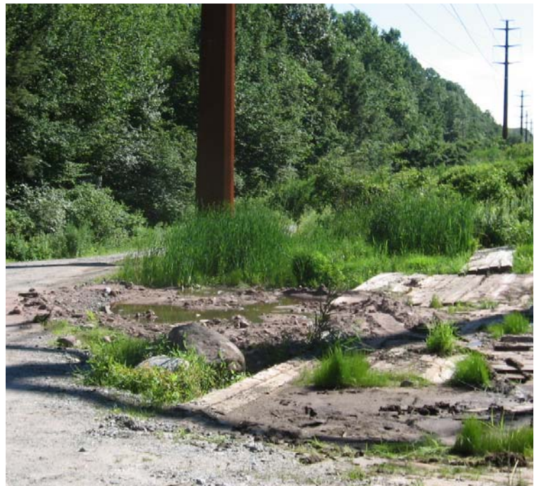
Gaylord Mtn Rd (Hamden): The spoil pile has been removed from the wetland near structure # 3992.
