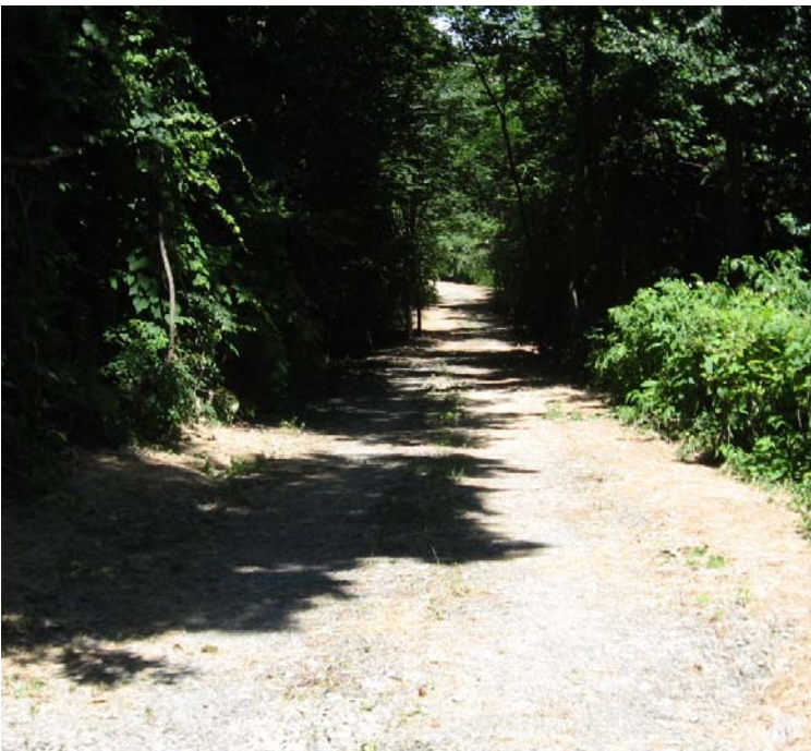
East Rutland: The access road to structures # 3827/24014 remains. Exposed soils have been graded and temporarily stabilized with mulch.
