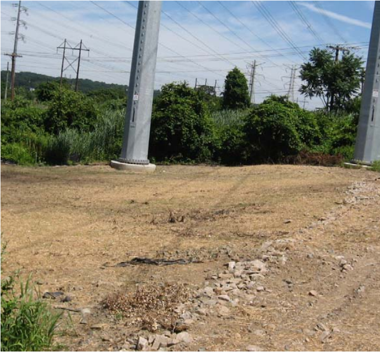
Naugatuck Rd (Milford): A view of 345 kV restoration efforts.
