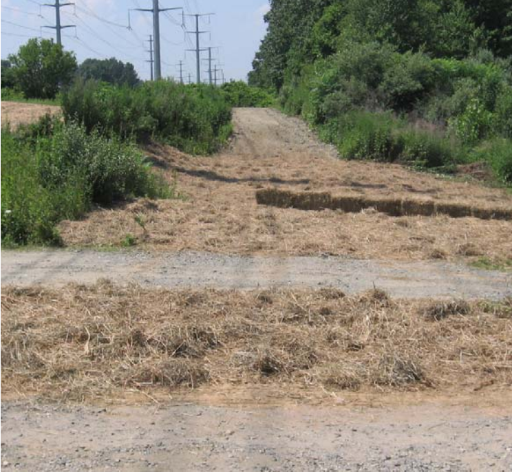
Oronoque Rd (Milford): A view of 345 kV restoration efforts.
