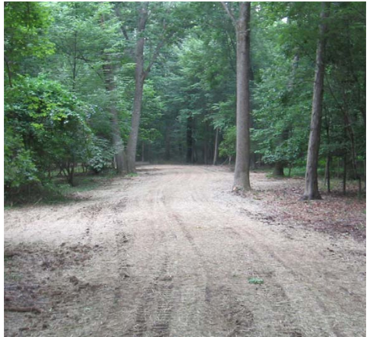
Clearview Ln: An additional view of upland access road restoration efforts.
