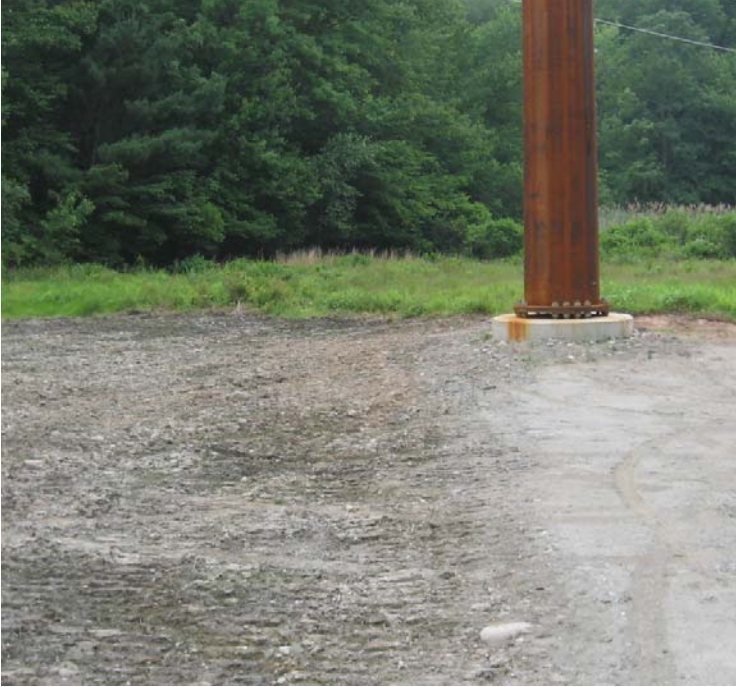
Clearview Ln: The stone crane pad was removed and soils were graded in the wetland area near structure #24086.
