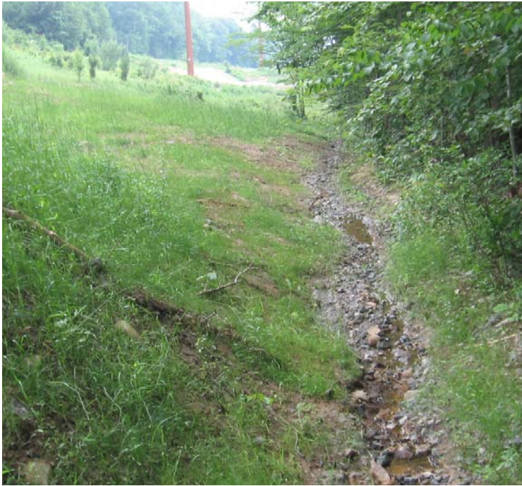
Gaylord Mtn Rd: An additional view of the vegetative swale.
