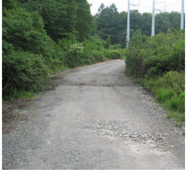
Clearview Ln: The access road to structures #3899/24086 is located within a wetland. The road has been graded and a waterbar was installed to allow water flow.
