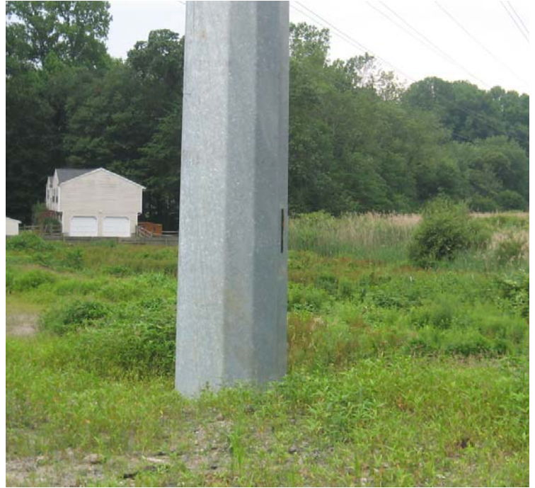
Oronoque Rd: A view of vegetative growth and 115 kV restoration efforts.
