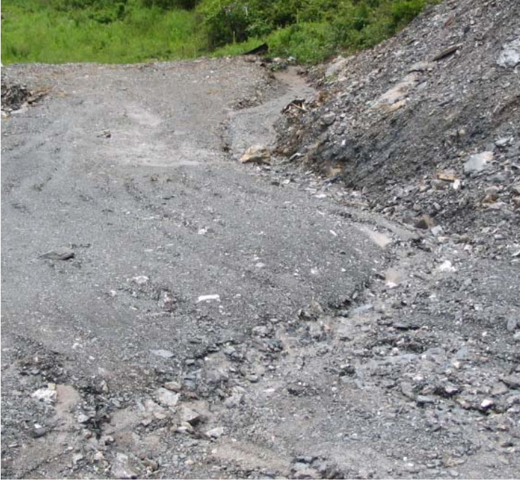
Litchfield Turnpike: An additional view of the waterbar and sediment basin near structure #24148.
