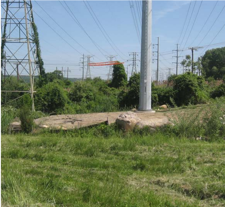
Naugatuck Ave (Milford): Wetland timber mats remain in the wetland area near structure #3804.
