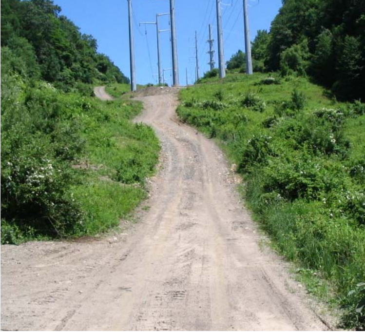
Glen Dam (Woodbridge): The access road, located on a steep slope, remains stable and stormwater controls remain functional.
