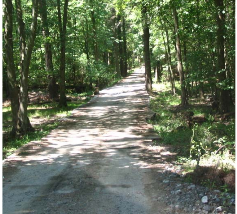
Clearview Ln (Woodbridge): The timber mat crossing remains in the wetland here.
