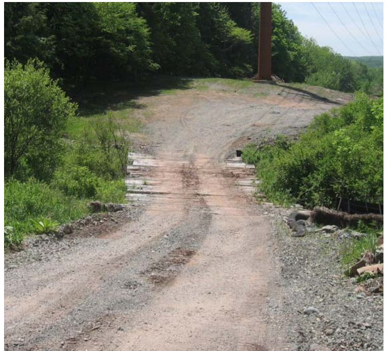
Old Ln: A view of the access road controls located at the base of the slope. Wetland timber mats remain in this area.
