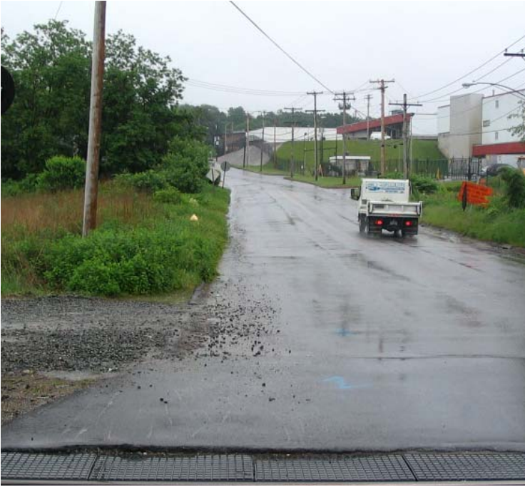
Caswell St (Milford): View of the northern access road entrance. Some sediment tracking was observed on Caswell St this week.
