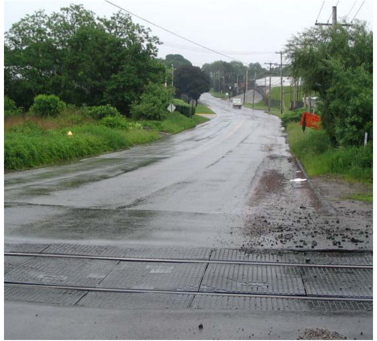
Caswell St: Sediment tracking was observed at the southern access off Caswell St.
