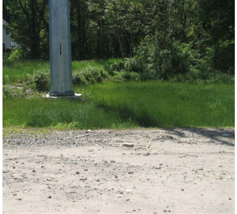
North St (south): A view of 115kV restoration efforts near structure #3844.
