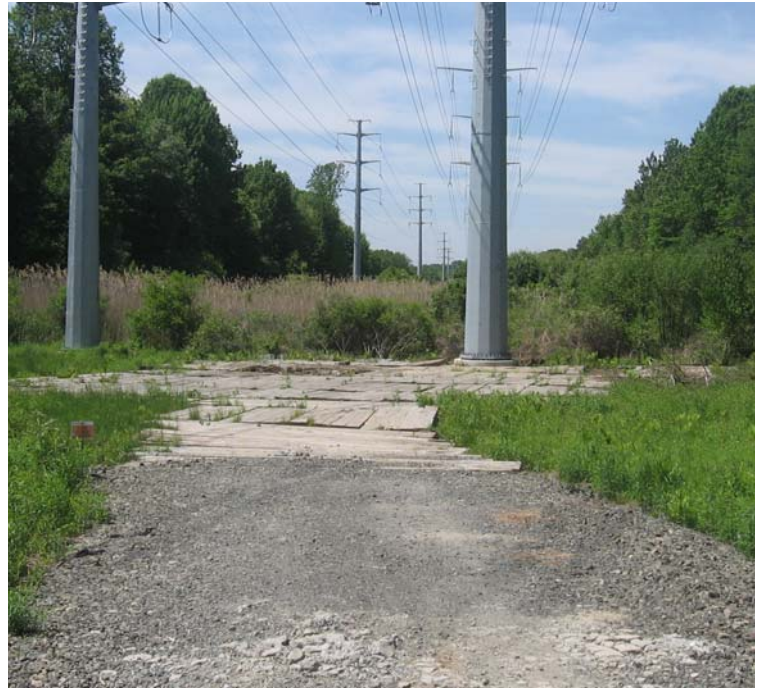
North St south: Timber mats remain within the wetland area here.
