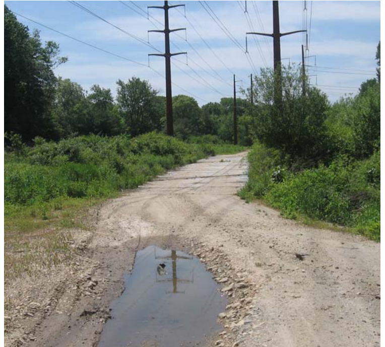
Sunset Dr (Orange): Timber mats remain within the wetland area here.
