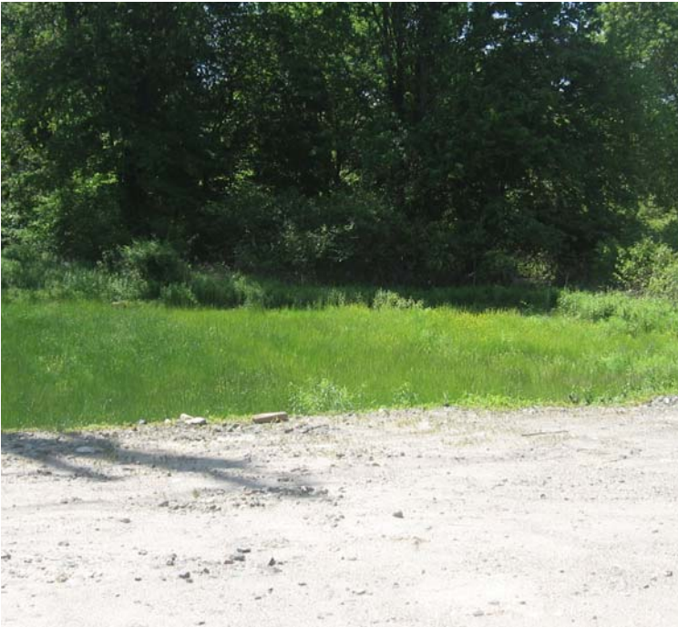
North St (south): An additional view of 115kV restoration efforts near structure #3844.
