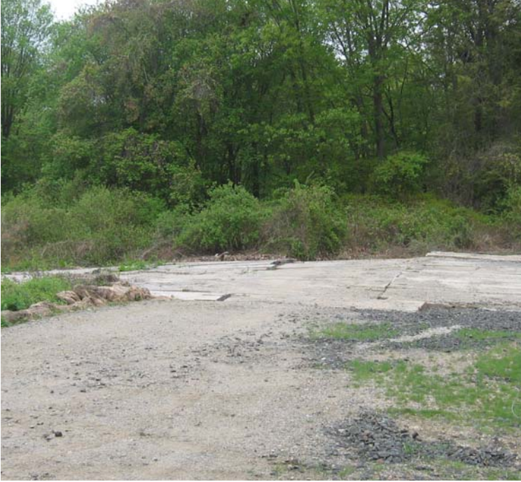
Eisenhower Park (Milford): Wetland timber mats remain near structure #3839/24026.
