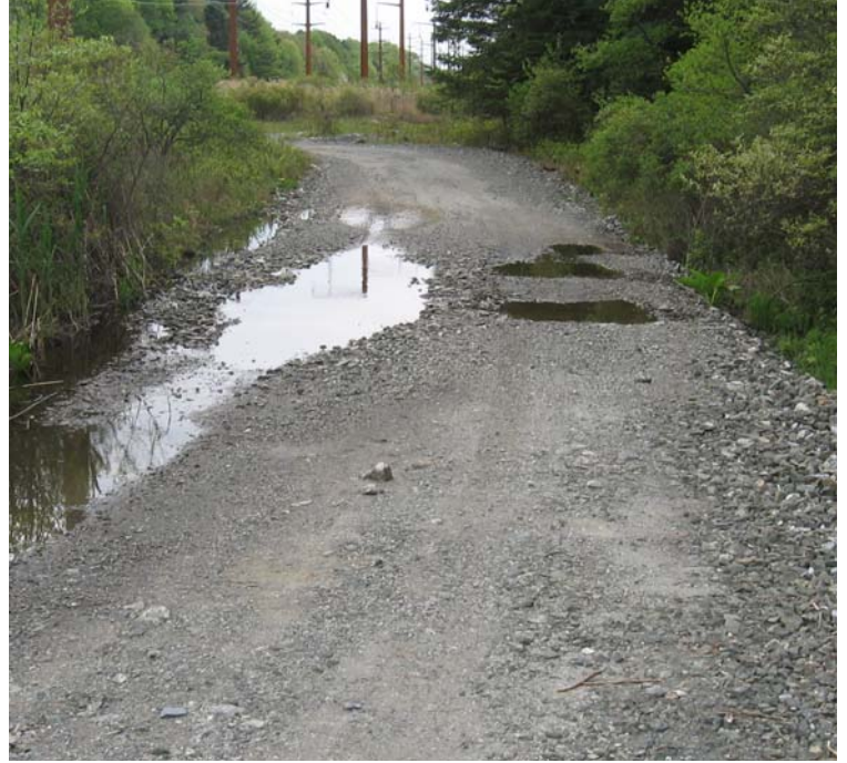
Clearview Ln (Woodbridge): The access road to structures #3899/24086 is impeding water flow from the eastern portion of wetland to the western portion.
