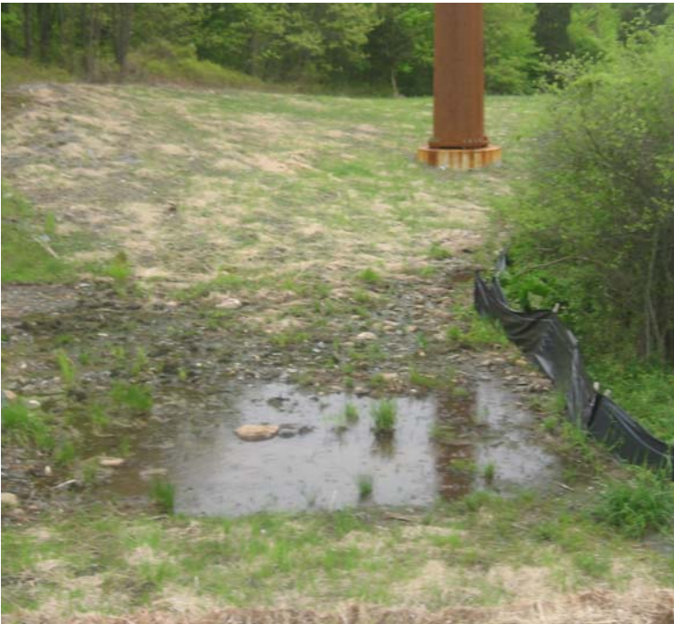
Litchfield Tpk (Bethany): A view of 115 kV restoration efforts at structure #3961.
