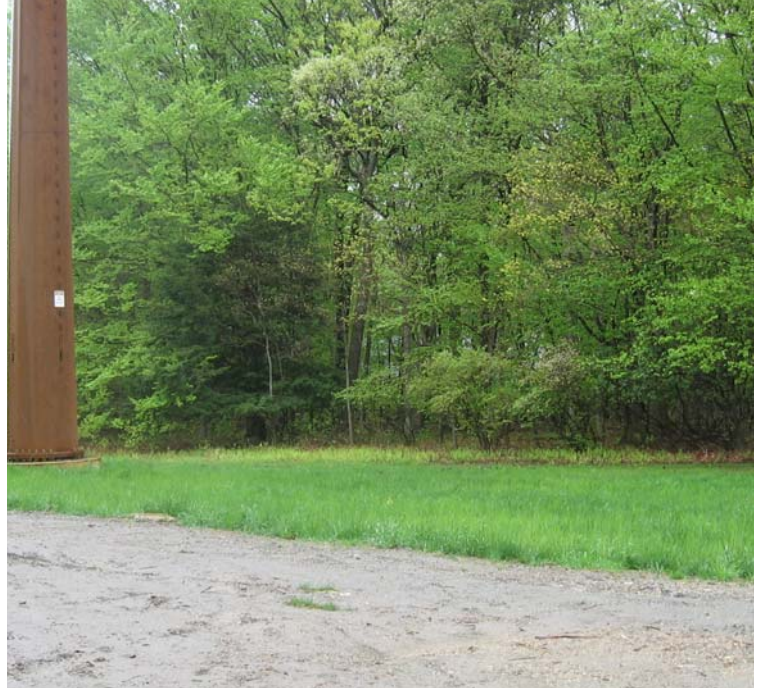
Pine Tree Dr: A view of 115 kV restoration efforts near structure #3857.
