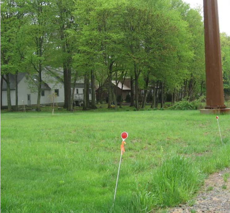
Pine Tree Dr (Orange): A view of 115 kV restoration efforts near structure #3855.
