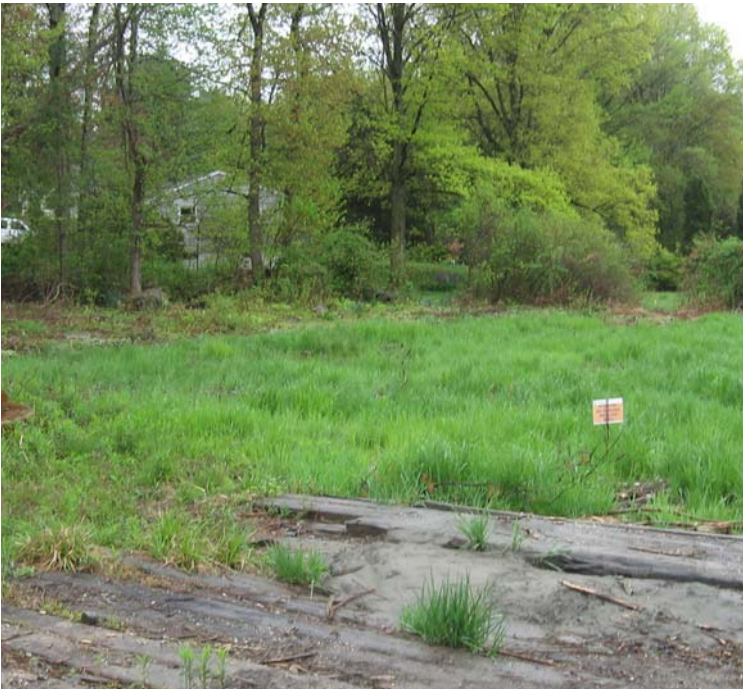
Racebrook Rd (Orange): A view of 115 kV restoration efforts near structure #3870.
