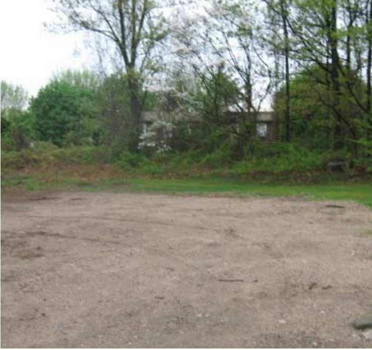
Plains Rd (Milford): A view of 115 kV restoration efforts at structure #3816.
