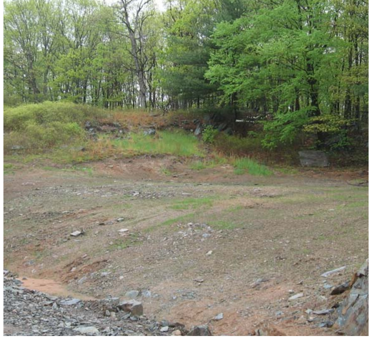
Rt 34 (Orange): A view of 115 kV restoration efforts near structure #3887.
