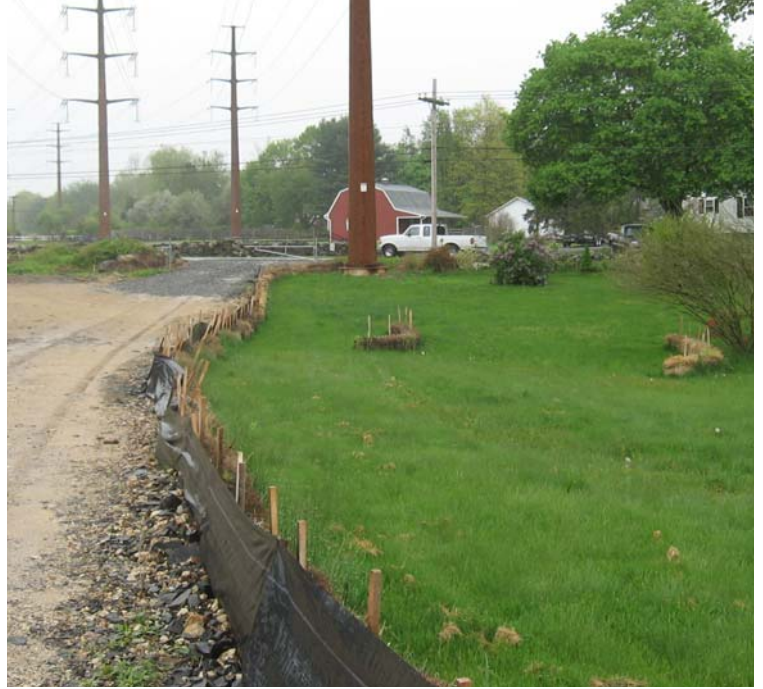
Ridge Rd (Orange): A view of 115 kV restoration efforts near structure #3848.
