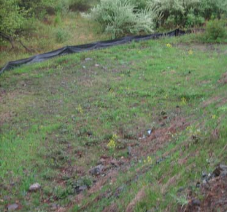
Lexington Way (Milford): A view of 115 kV restoration efforts near structure #3826.
