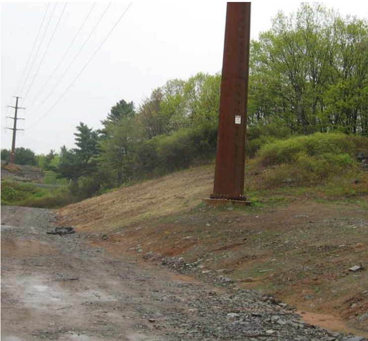
Rt 34: A view of 115 kV restoration efforts near structure #3887.
