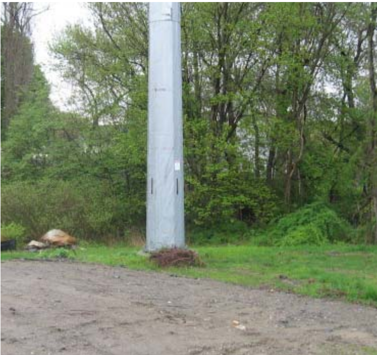
Oronoque Rd (Milford): A view of 115kV restoration efforts near structure #3821.
