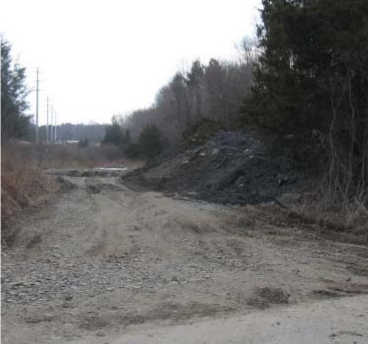
Brookwood Dr (Woodbridge): Stockpiling continues near structure #24096.
