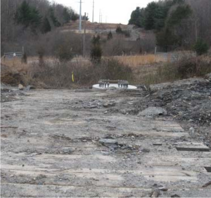
Morris Rd (Woodbridge): Structure #24146 has been installed within wetland #121.
