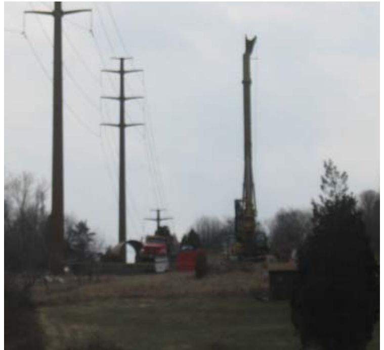
Saddle Ridge Rd (Orange): Drilling continues at structure #24071.
