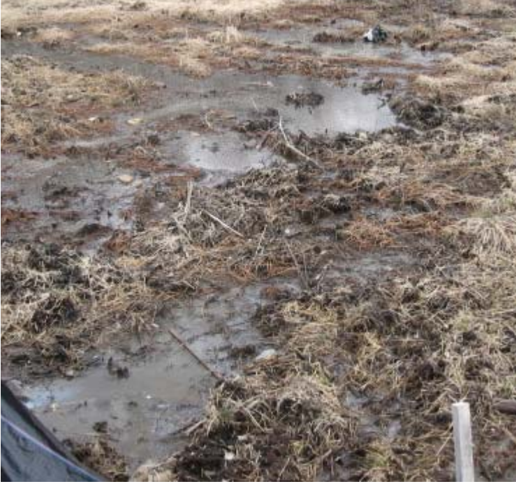
Manville Rd North (Woodbridge): An oily sheen was noted on the water surface near structure #24103.
