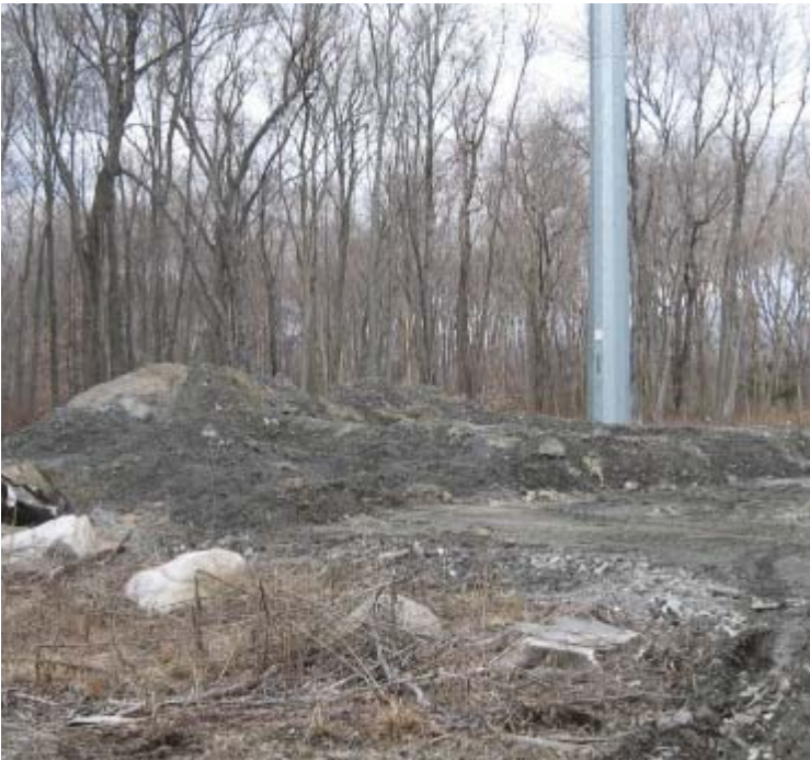
Pease Rd (Woodbridge): Stock piling continues near structure #24112.
