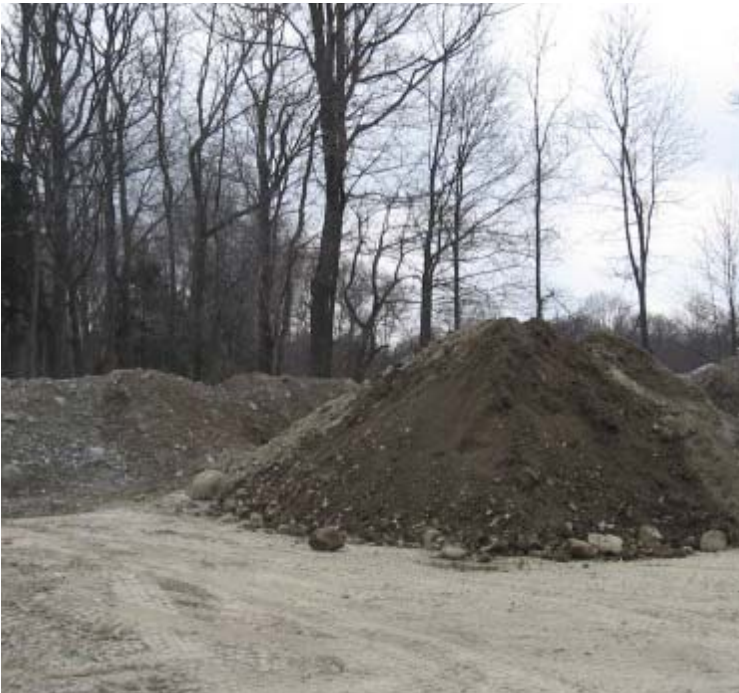
Dogwood (Orange): Stock piling continues near structure #3879.
