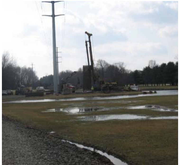
Oak Ln Country Club (Woodbridge): Drilling continues at structure #24093.
