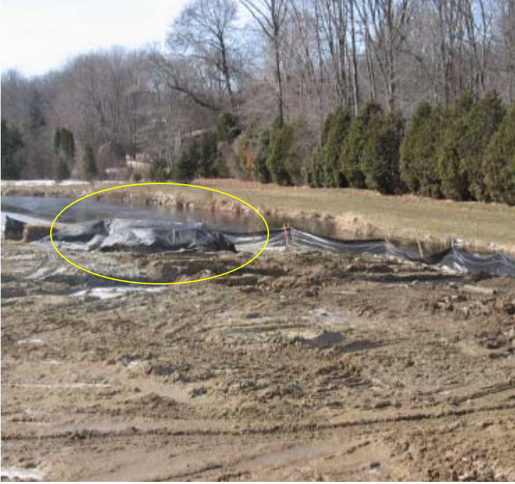
Dogwood Rd (Orange): Foundation installation appears complete at structure #24065.
