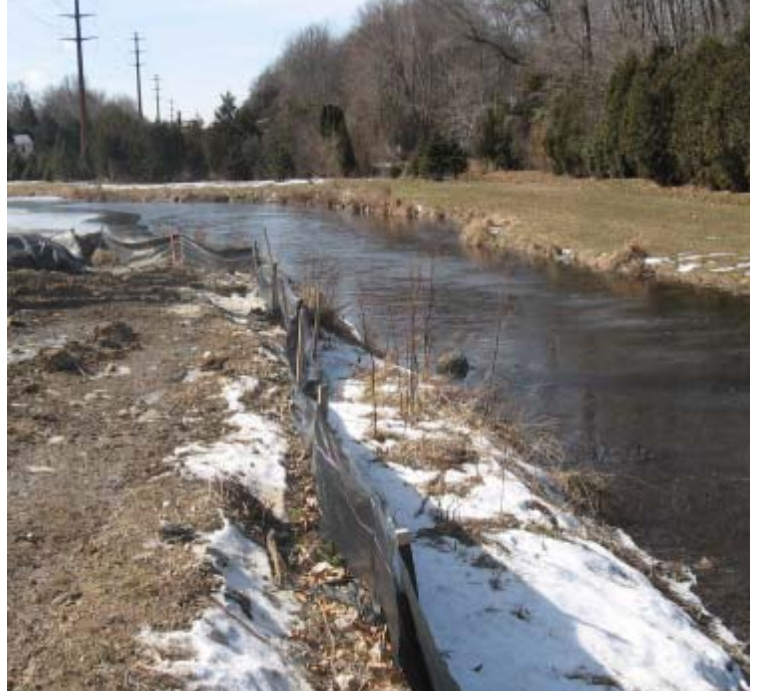
Dogwood Rd: Erosion controls are in place and functioning properly.
