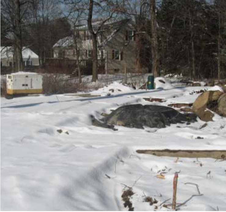
Racebrook Rd (Orange): Foundation installation appears complete at structure #24057.
