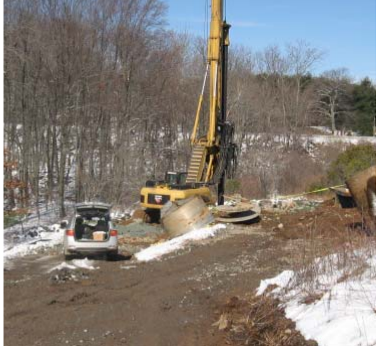
Route 34 (Orange): Drilling continues at proposed structure #24074.
