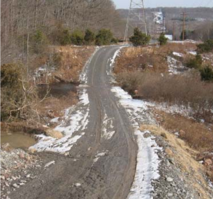
Brooksvale Ave (Hamden): Existing access controls remain functional, but additional controls are needed to help prevent sedimentation on the timber mat crossing and within the wetland.
