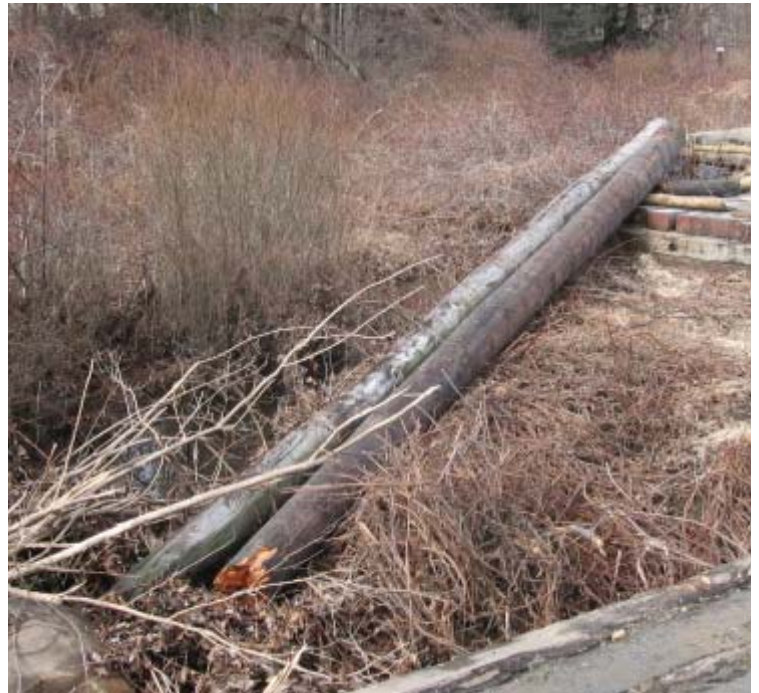
Rimmon Rd (Woodbridge): A disassembled "H-frame" structure remains in the wetland area here.
