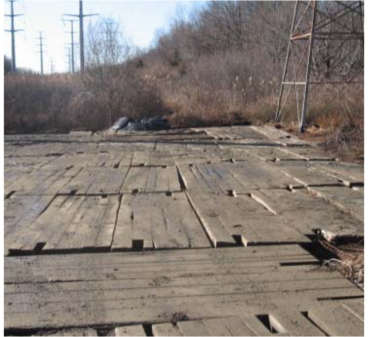
North St: Foundation installation is complete at structure #24032.
