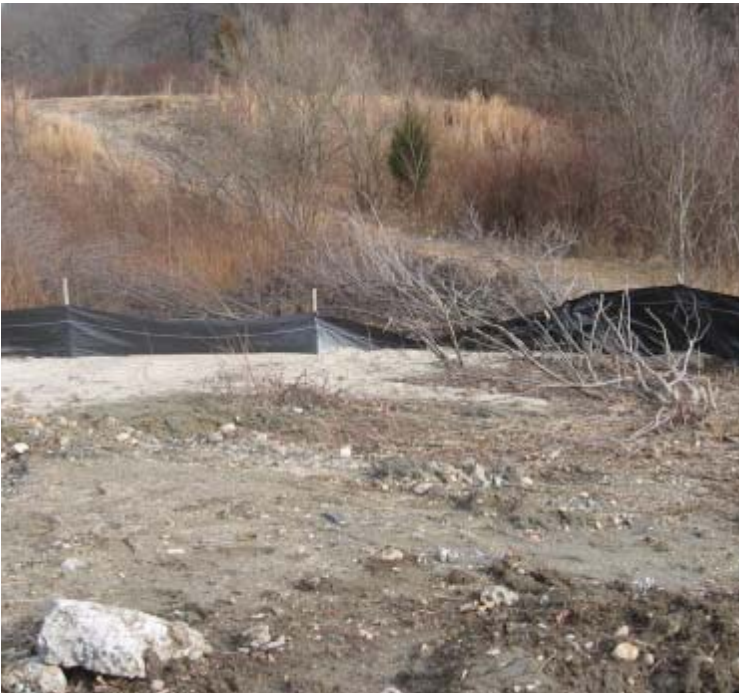
Eisenhower Park (Milford): Sand, used during foundation installation, is overwhelming the controls near structure #24027.
