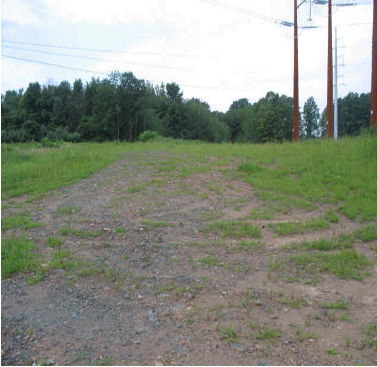
Carpenter Ln: The disturbed area remains graded and seeded but vegetative growth is still fairly sparse. Additional seed may be needed during more favorable conditions.
