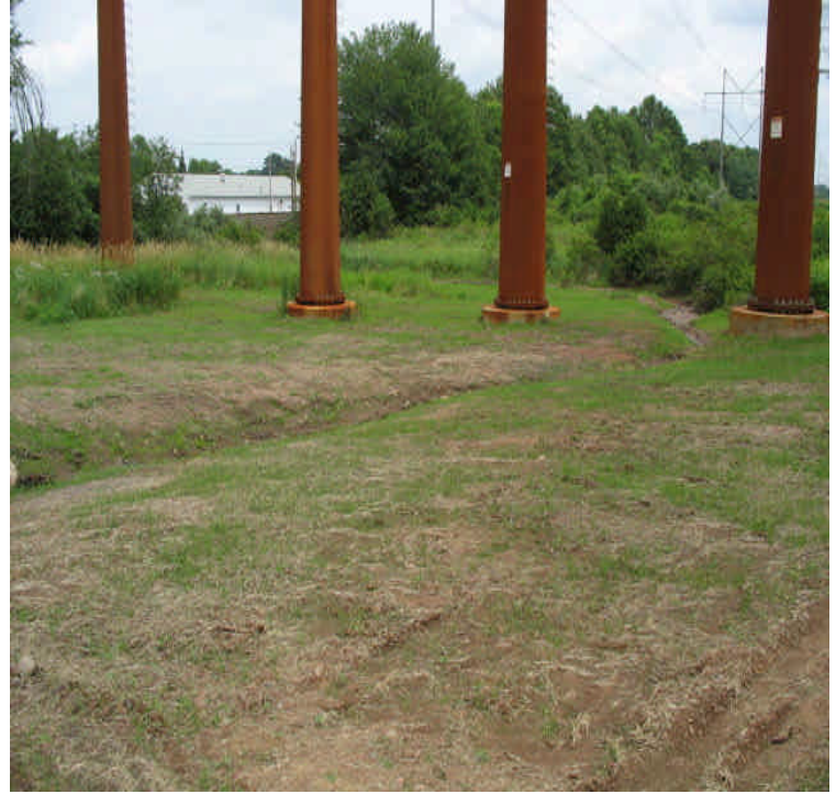
Powers Rd: Final restoration complete. Some grass growth noted. Additional seed may be needed along the banks if vegetation remains sparse.
