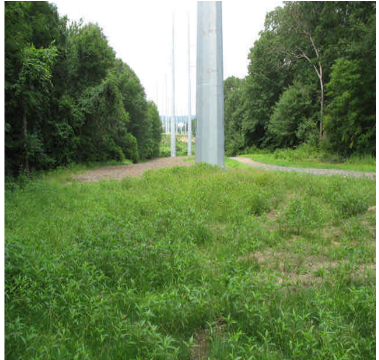
Docker Dr: Vegetation was establishing due to reduced ATV use. Bark mulch along the slope is holding up well.
