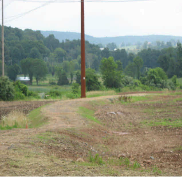
Tamarack Swamp Rd: Access road pads narrowed and graded.
