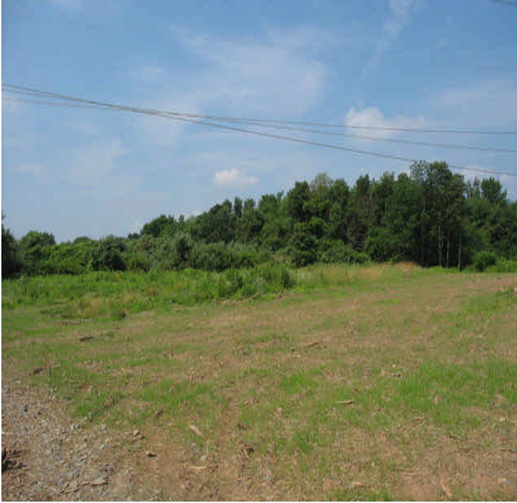
Carpenter Ln: Soil stockpiles were removed and the disturbed area has been graded and seeded. Some grass growth was noted.
