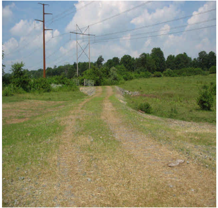
Tamarack Swamp Rd: Final restoration complete. Some grass growth noted.
