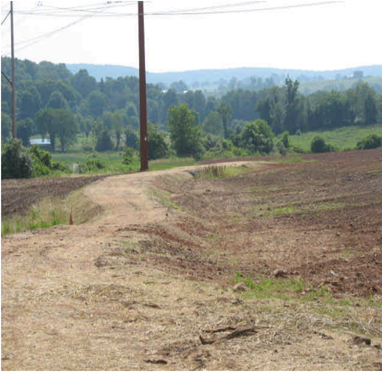
Tamarack Swamp: Access road pads narrowed and graded.
