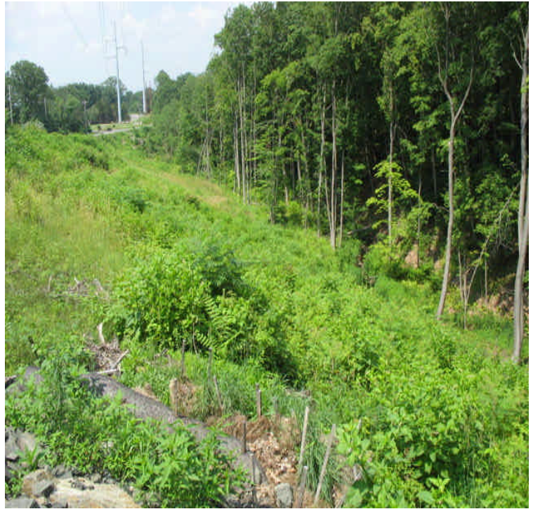
Harrison Rd: Re-vegetation continuing along the ROW from Woodhouse Rd. This steep slope is also stable.
