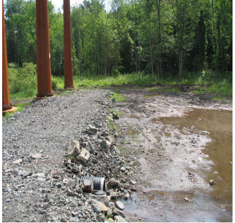
Carpenter Ln: Restoration work is complete within the wetlands. Minor seeding will be done when water subsides. Impacts were reduced from original permitted numbers and narrowed to a spur road.
