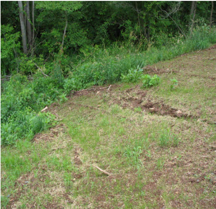
Durham Rd (North): Small gully was noted from recent storm event. Regrade and monitor for stabilization.
