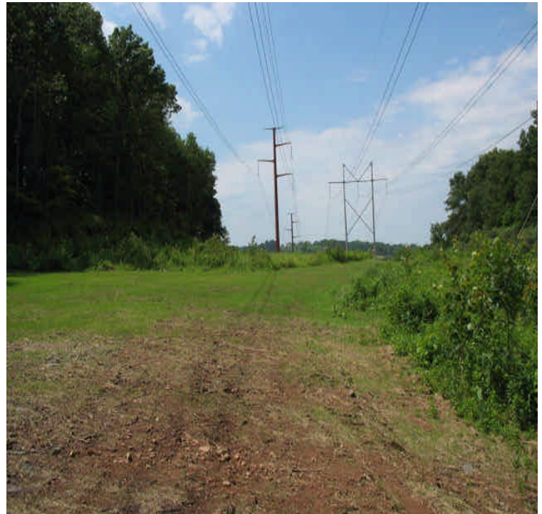
Stony Brook: Final grading/restoration complete. Topsoil, hay and seed have been spread.
