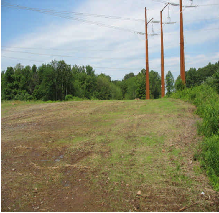
Carpenter Ln: The disturbed area upgradient of wetlands remains graded and seeded with some new grass growth.
