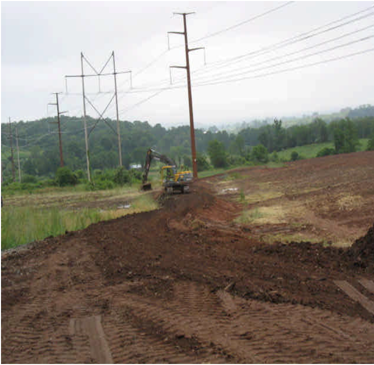
Tamarack Swamp Rd: Access road pads being narrowed and graded.
