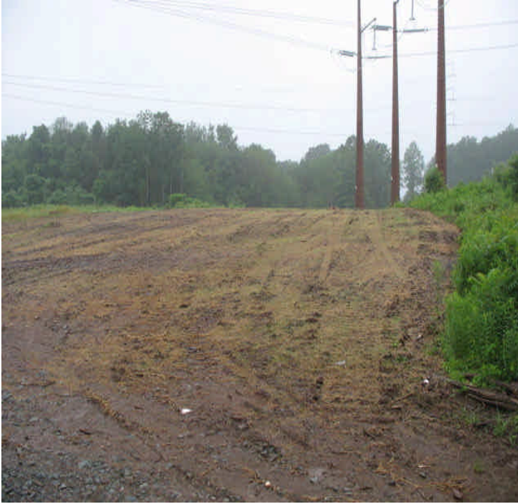
Carpenter Ln: Soil stockpiles were removed and the disturbed area has been graded and seeded
