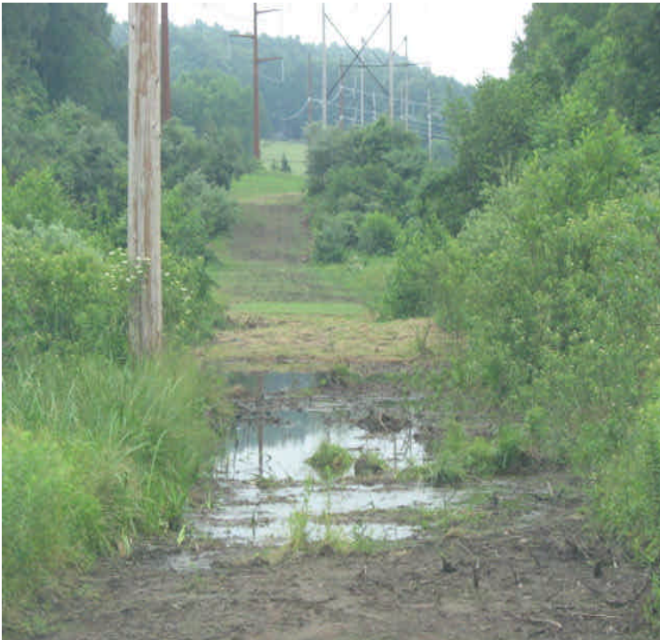
Durham Rd (south): Exposed soils from Durham Rd south need to be stabilized. Controls upgradient of the wetlands are needed.
