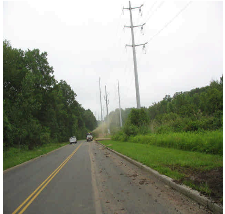
Old Farms Rd: Sediment tracking from the restoration efforts. Clean/sweep roadway as needed.
