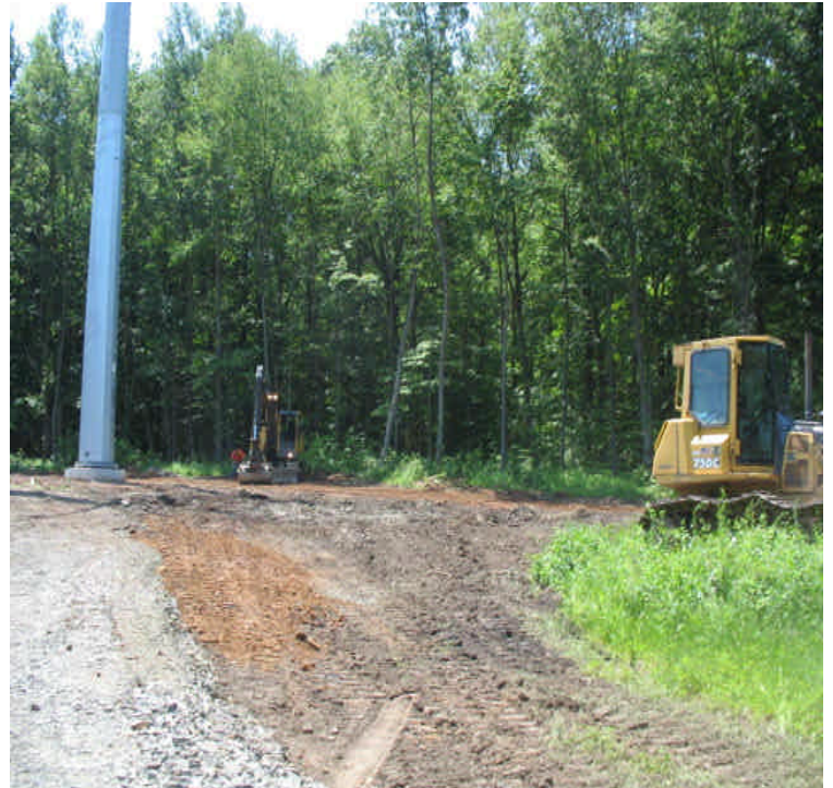
Mansion Rd: Final restoration/reclamation underway.
