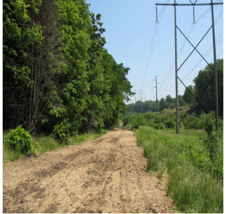
Liney Hall: Timber mats and bridge were removed. Hay and seed were applied up to the gated access to the adjacent property.
