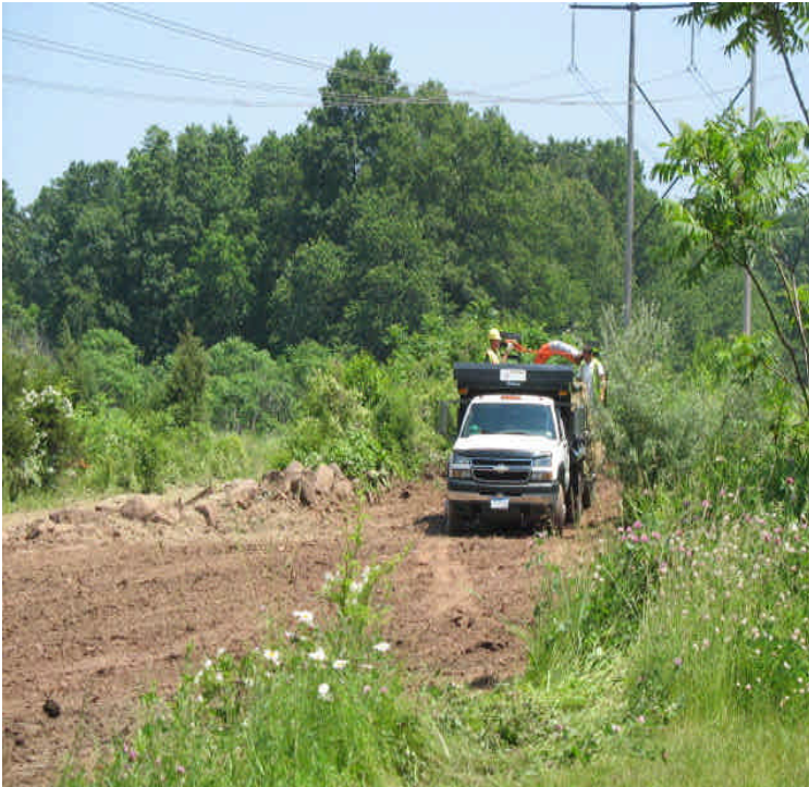
Stony Brook Rd: Crews were spreading hay and seed on exposed areas.
