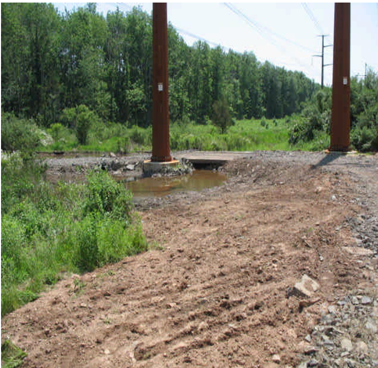
Carpenter Ln: Final restoration complete. Monitor exposed soils upgradient from wetlands.
