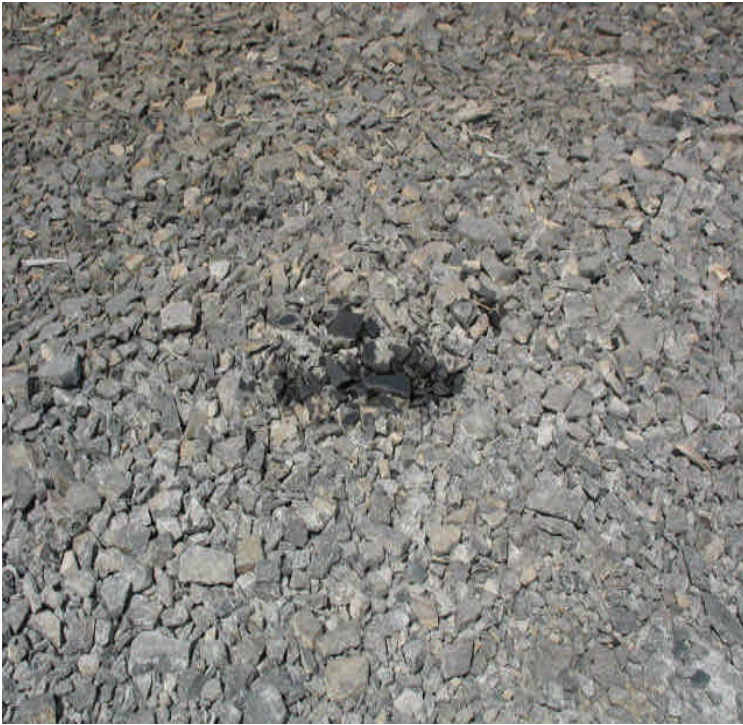
Stony Brook Rd: Hydraulic fluid drips noted at the site entrance. Crews were working to check and repair the leaking equipment.
