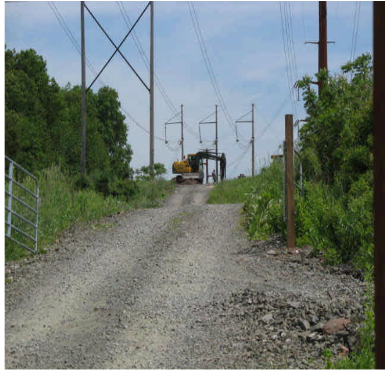
Stony Brook Rd: Final restoration continues.
