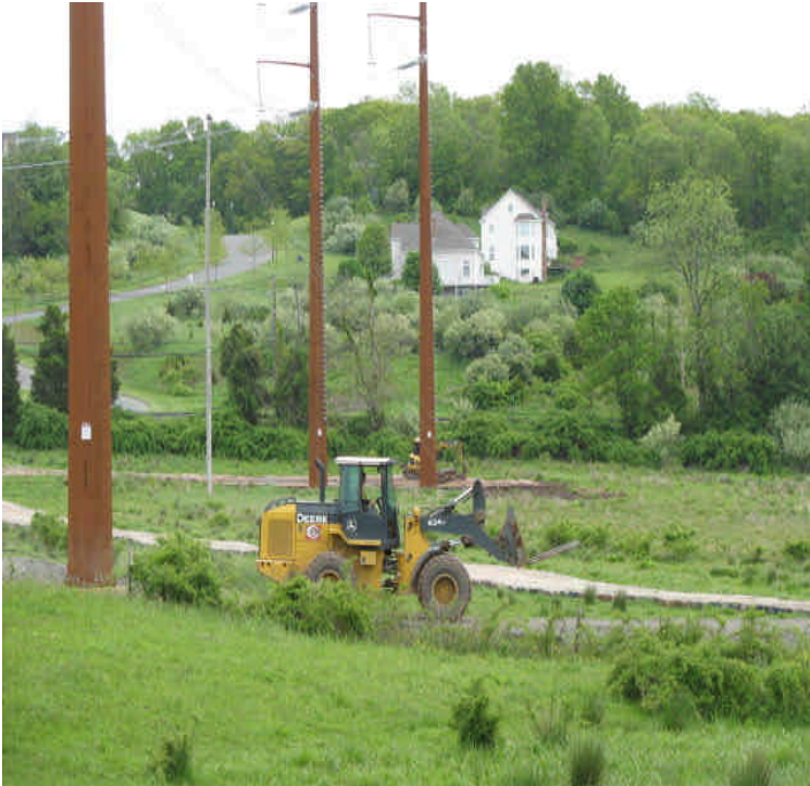
Tamarack Swamp Rd: Timber mat removal underway within wetlands.
