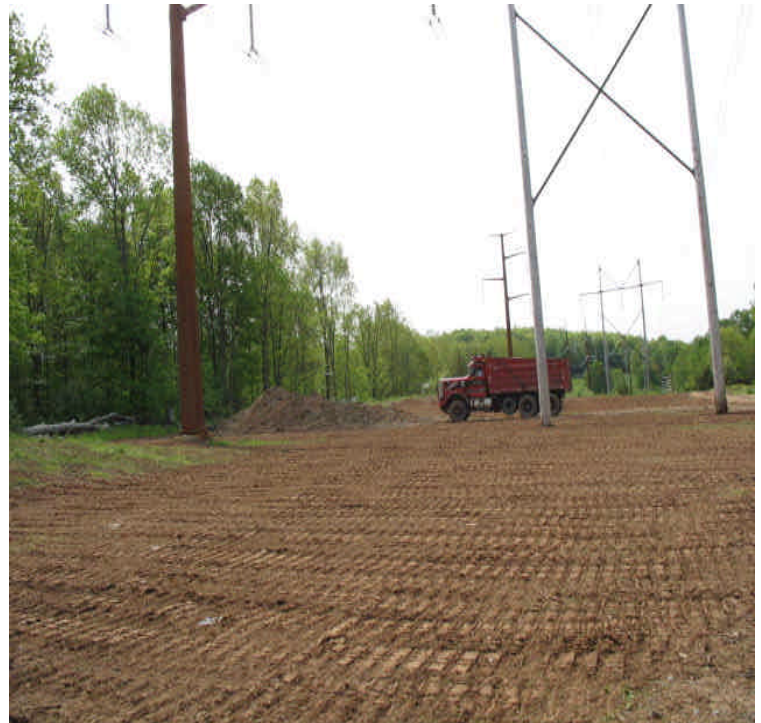
Durham Rd: Final grading/restoration was underway.
