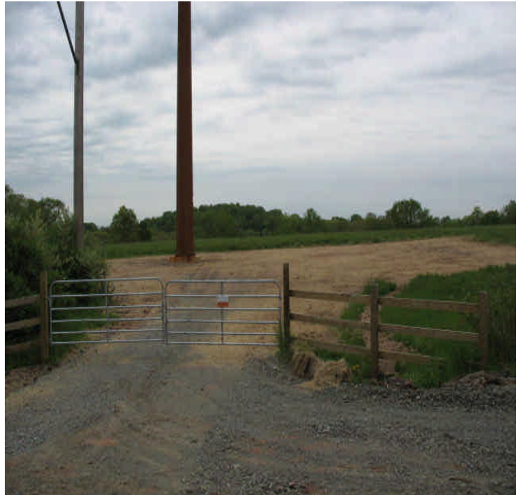
Tamarack Swamp Rd: Stockpile has been removed and crews had just completed application of mulch and seed.
